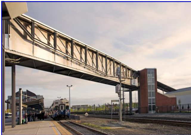
Everett Station Pedestrian Bridge
