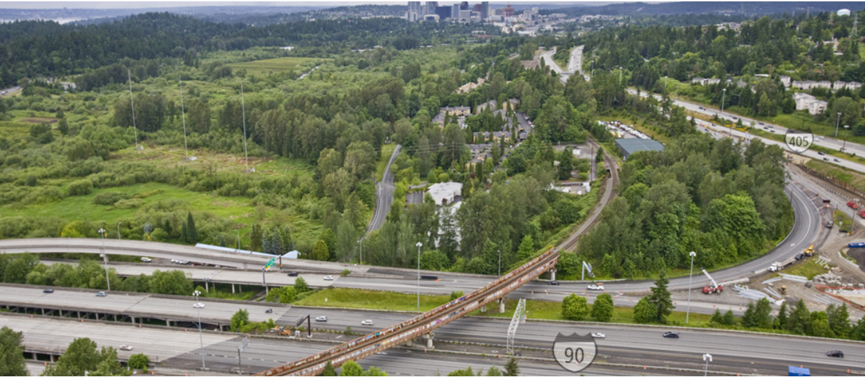
Burlington Northern Santa Fe (BNSF) Eastside Corridor crossing I-90 south of downtown Bellevue
