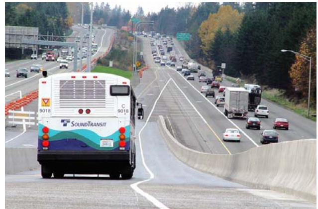
BRT= Bus Rapid Transit is a system of frequent bus service operated in dedicated running ways or HOV lanes.
