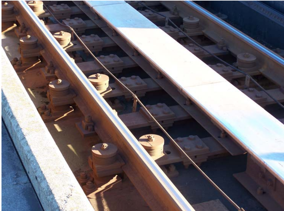
Photo 3: Close up of the vertical movement mechanism of the rail joint
