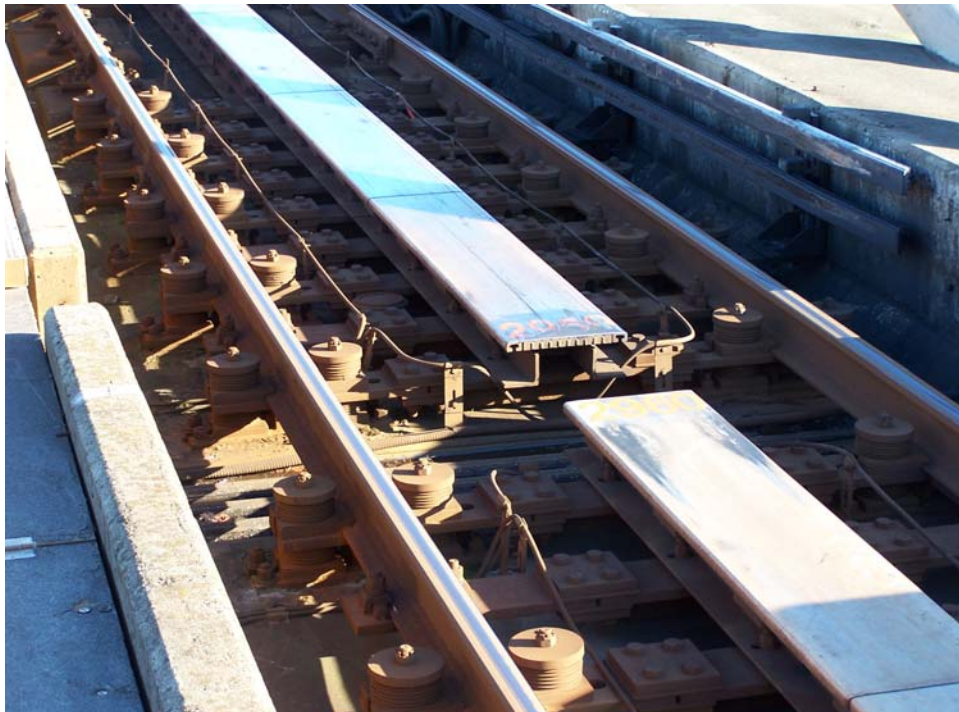
Photo 4: Close up of the bridge transition section
