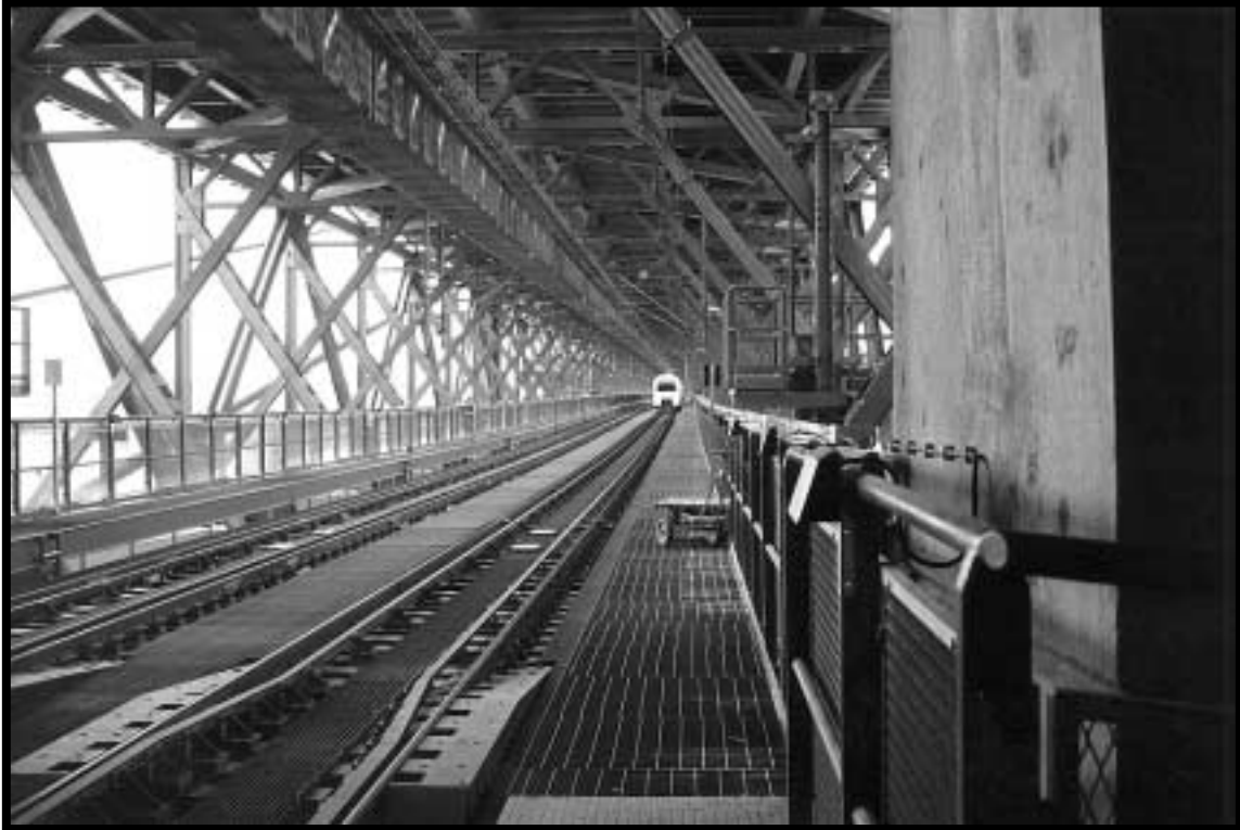
Photo # 7 - View of Double Track at Ends
