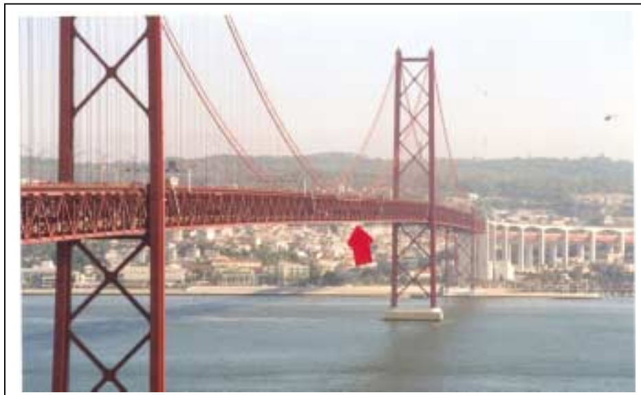
Photo #2 - Deflection during passage of train
