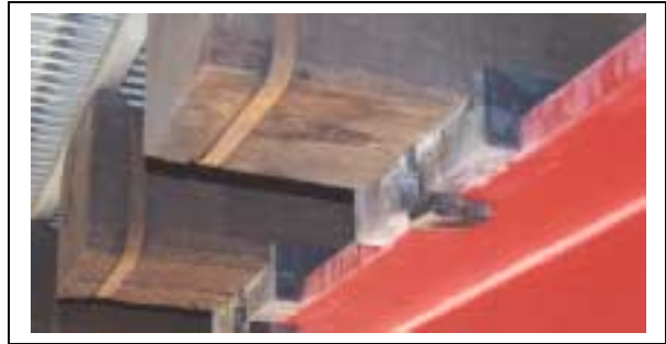
Photo #4 - Hook Bolt and Plastic Pad as seen from bottom
