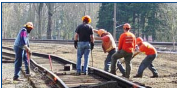
Workers relocate rail tracks
