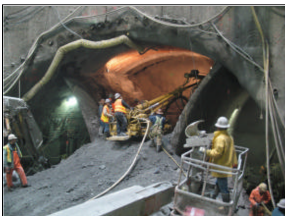
Mining the station's underground concourse
