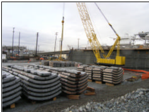
Pre-cast tunnel liner segments at the west portal
