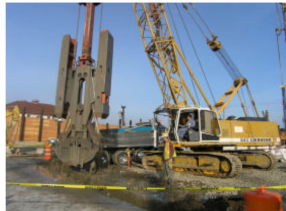
Digging the underground wall for the station
