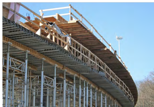
Construction of Elevated Guideway Showing False-Work
