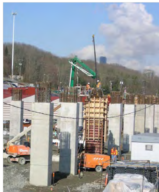
Columns Under Construction for the Central Link Project in Seattle
