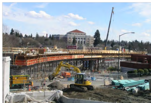
Staging Area Adjacent to New Guideway Under Construction
