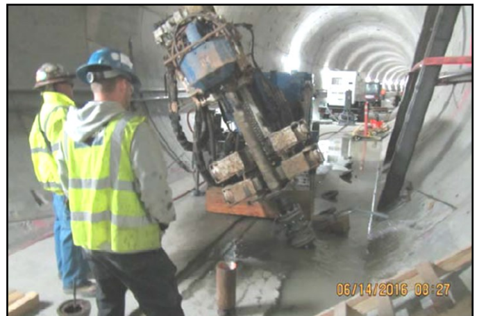
Drilling in-tunnel haunch freeze pipes in NB tunnel of CP34.
