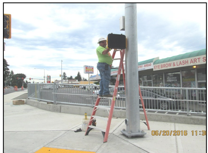
Installing pedestrian signals at the corner of S200th and 28th.
