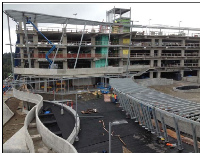
Structural framing of plaza canopy nearing completion.
