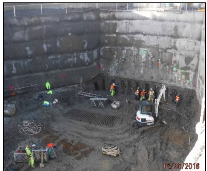
Preparing headwall for shotcrete.
