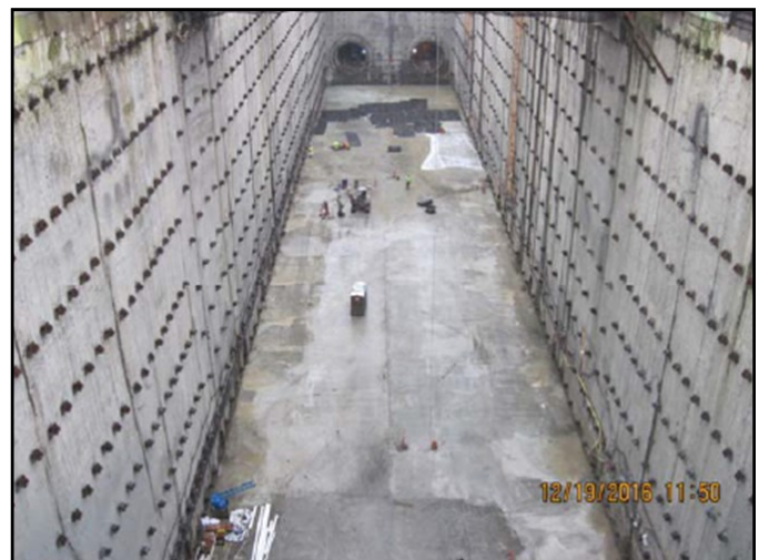
Completed permanent rat slab for the entire RVS station box.
