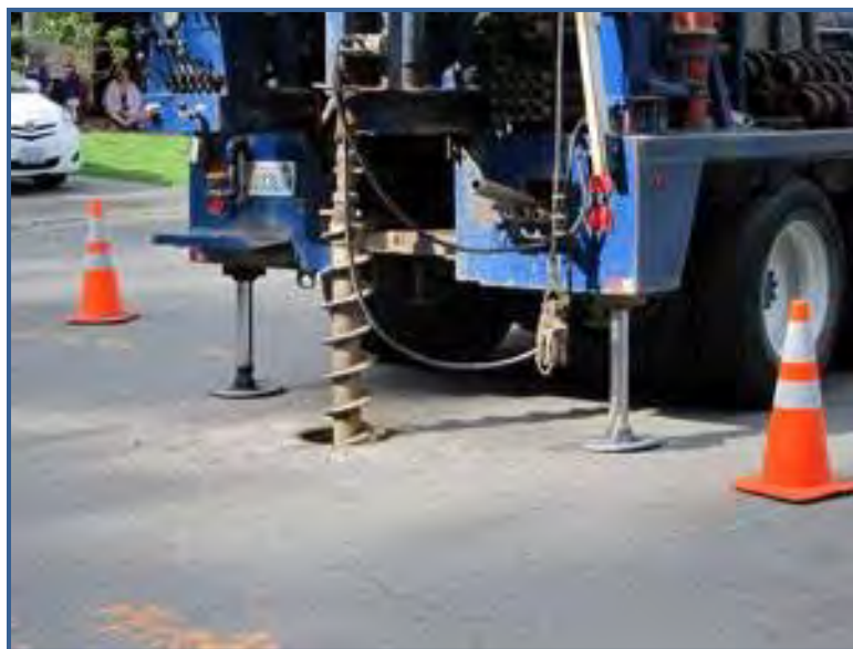
Geotechnical drilling in Mountlake Terrace as part of the environmental review process for Lynnwood Link Extension
