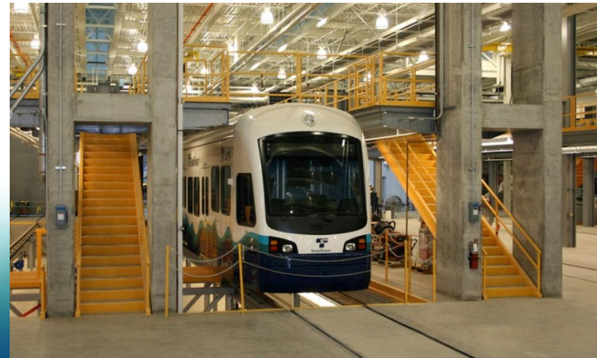
OMF Shop and Service Bays
