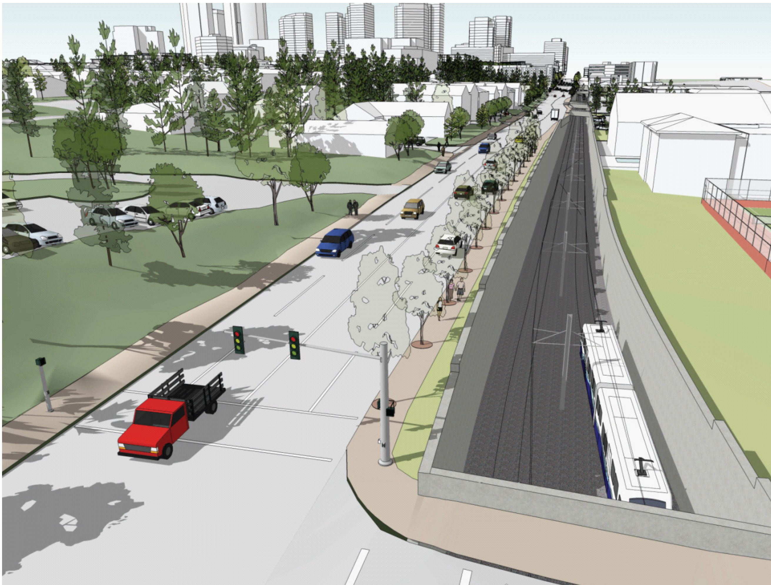
112th Ave SE at SE 6th Street: Retained Cut
