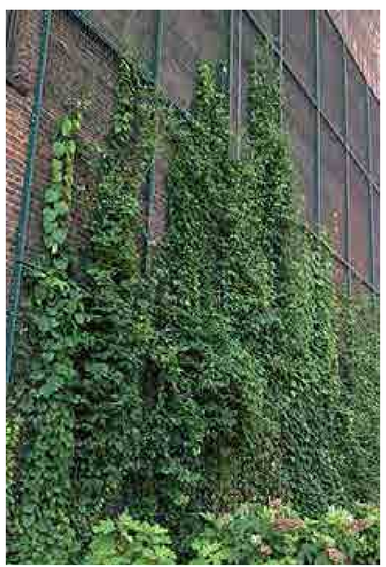
Mesh Wall Screen Coated metal mesh panels support twining vines desirable to cover walls.
