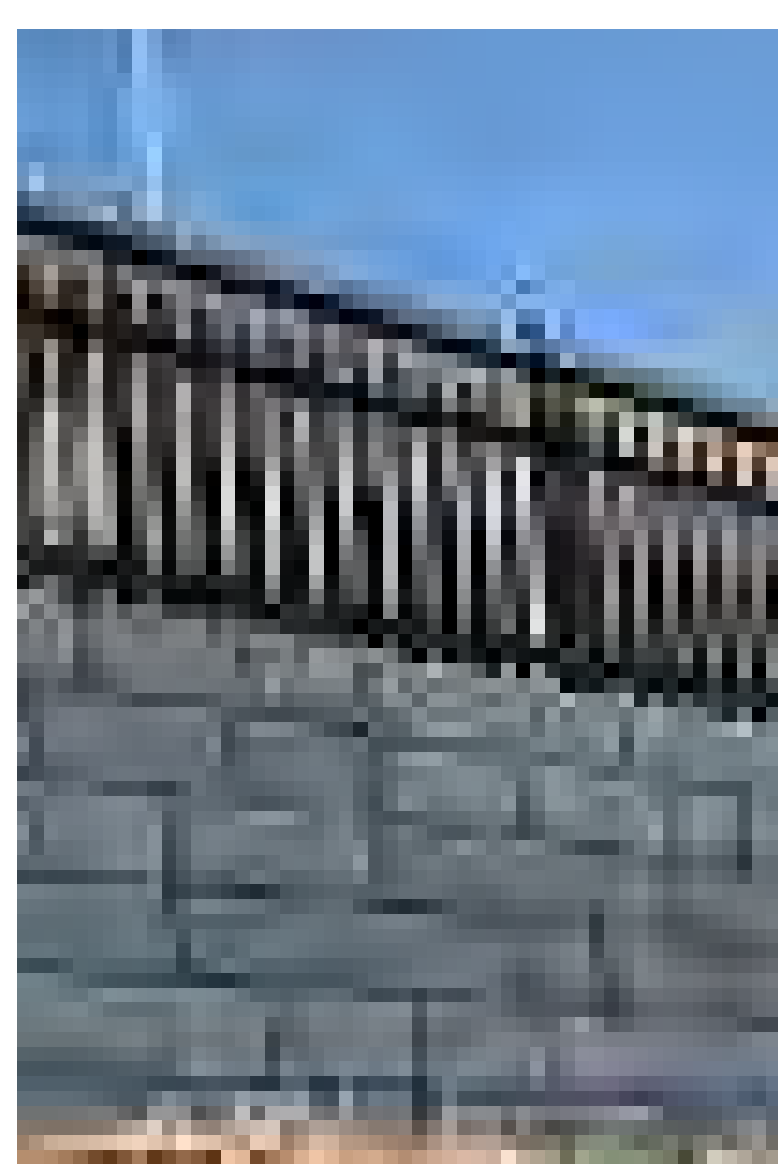
Fabricated Metal Guards on Wall to match Station accessories Guard with graspable railing positioned on top of low wall to protect and buffer pedestrians from parking lot adjacent to trail.
