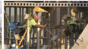
Sound Transit Civil Construction Approximately 3 years of phased work
