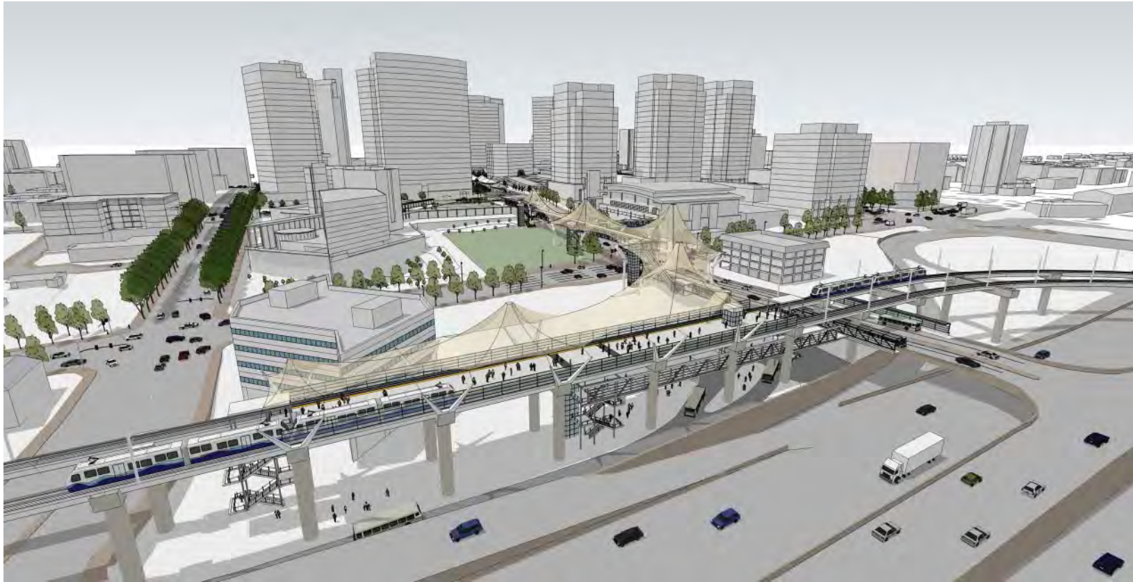
C14E: 114th NE Elevated Alternative – Station at 114th Avenue NE Looking Northwest with Cover Shown as Transparent
