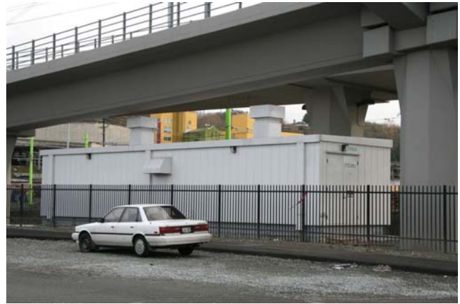
EXHIBIT 2-51 Traction Power Substation
