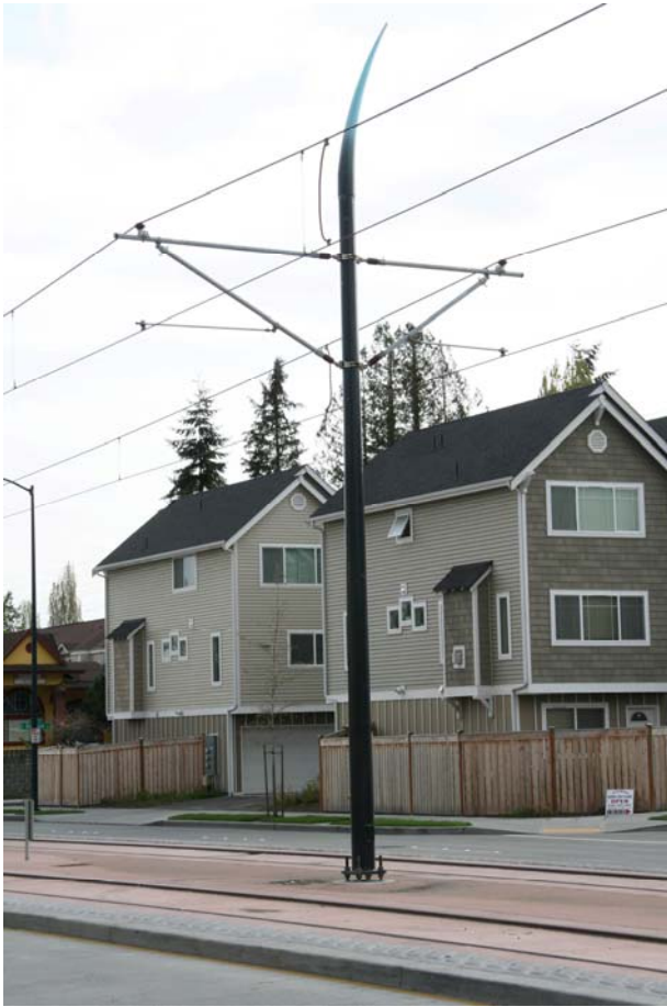
EXHIBIT 2-50 Overhead Catenary System
