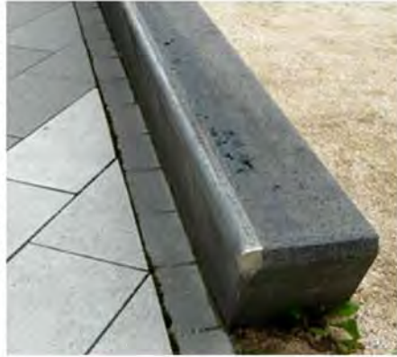
LANDSCAPE CURB WALLS
