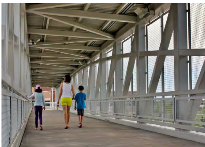
EXAMPLE OF PEDESTRIAN BRIDGE
