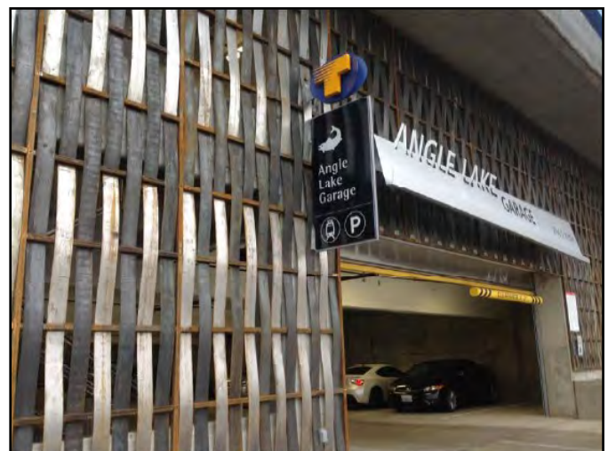
Installed overhead garage sign.
