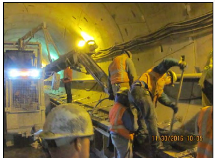
Pouring NB tunnel walkway concrete between UDS and RVS (CP29 to CP30).
