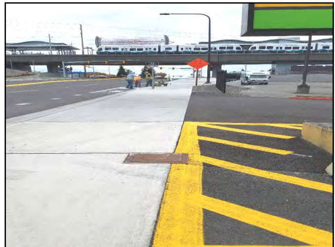
Adding bike lane markings on S. 200th.
