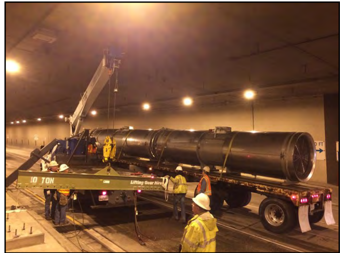
South Portal pipe canopy head wall in cut-and cover.
