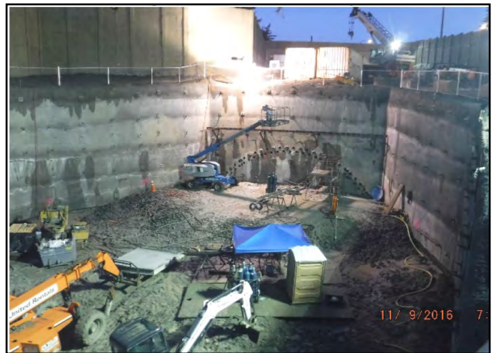
South Portal pipe canopy head wall in cut-and cover.
