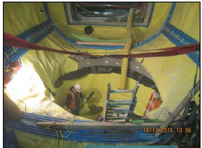
Completing drainage sump waterproofing at CP31.
