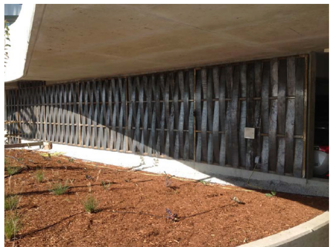
Completed decorative woven screen on south façade.
