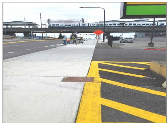
Adding bike lane markings on S. 200th.
