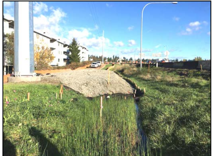
Review of MSE wall location, Pole Site 1. (Looking North)
