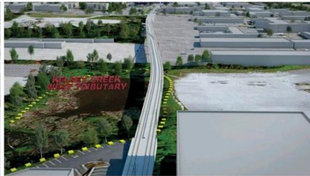
Aerial guideway over Kelsey Creek West Tributary, looking east (60% final design)
