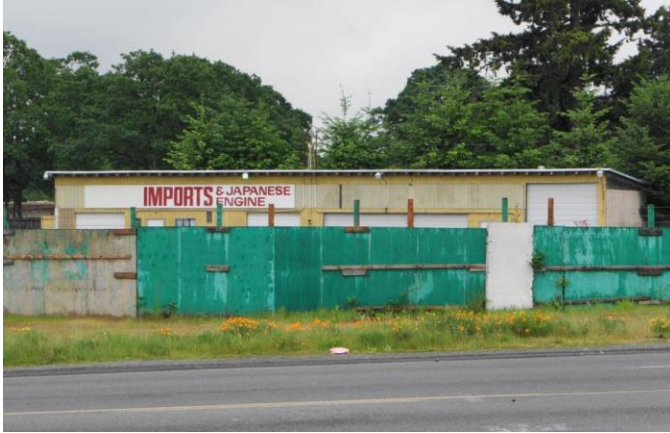
4046 100th Street SW Warehouse 2, north elevation 2013
