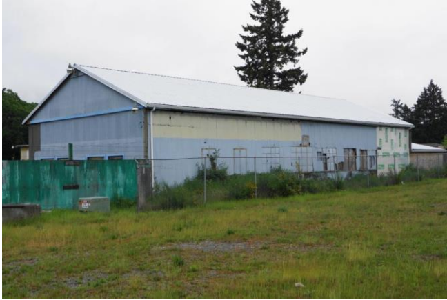
Warehouse 1, oblique of north and west elevations 2013
