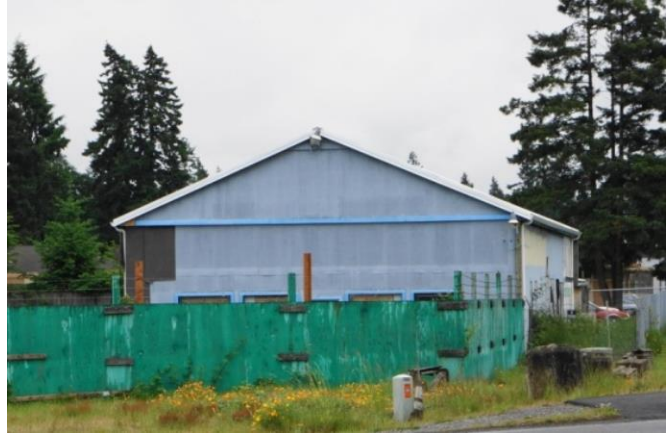
Warehouse 1, north elevation 2013
