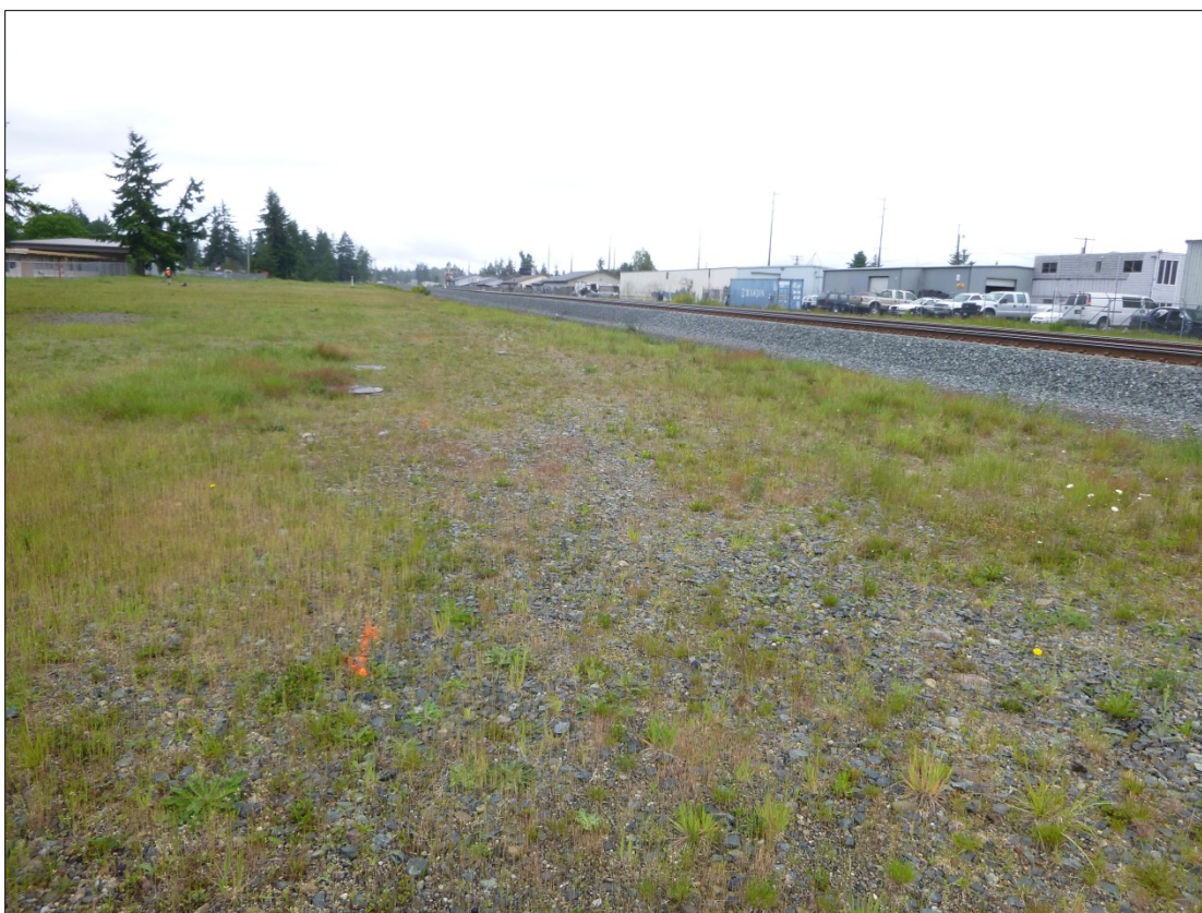
Figure 7-4 Overview of northern portion of Potential Future Project area (view south); note orange paint marking fiber optic line.
