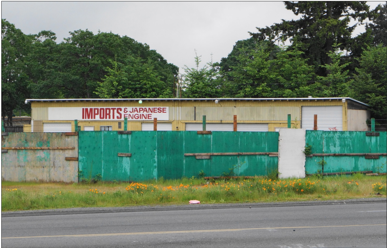
Figure 8-2. Lakes Auto Wrecking Warehouse #2 north elevation, 2013.
