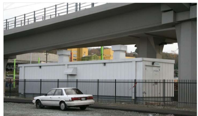
EXHIBIT 2-6 Traction Power Substation
