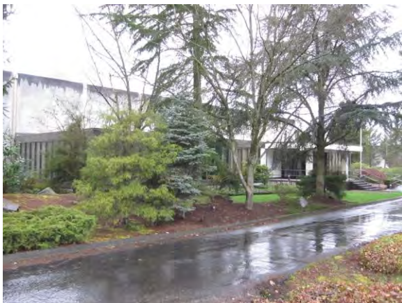
East Elevation, Looking Northwest 2013
