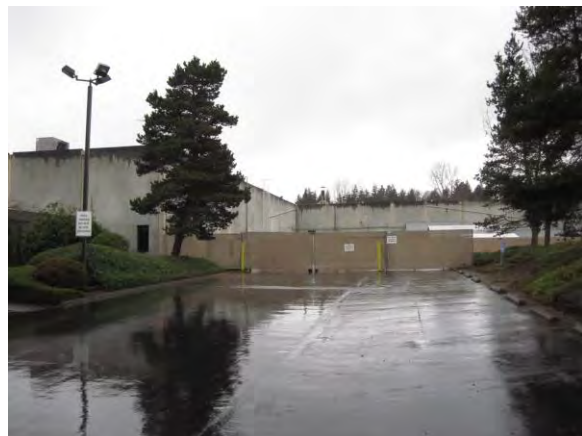
East and North Elevation, View West 2013
