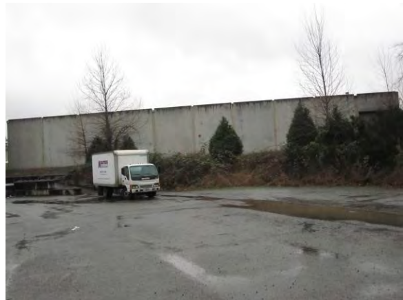
North Elevation, Looking South 2013
