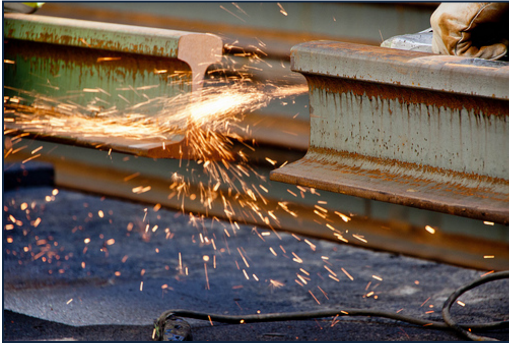
Capitol Hill Station Rail Construction
