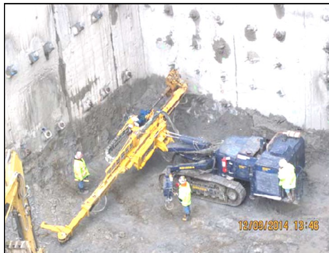
Test coring jet grout block for the NB tunnel eye location at RVS.
