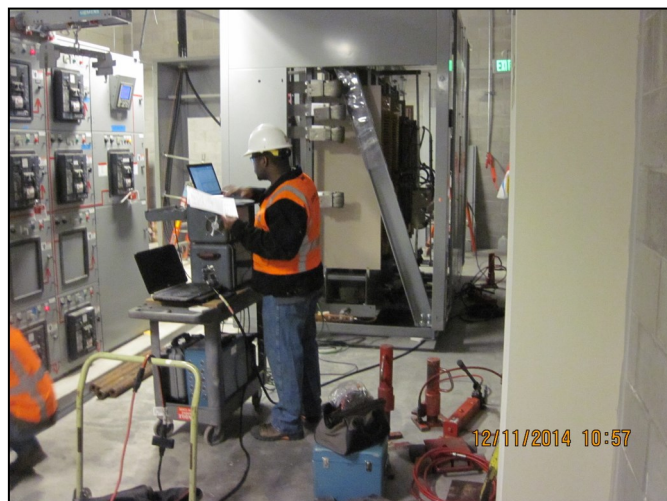
Testing transformer #2.
