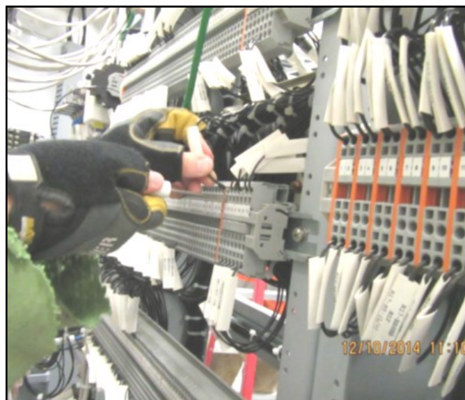
Rack wiring at the UWS Signal Room.
