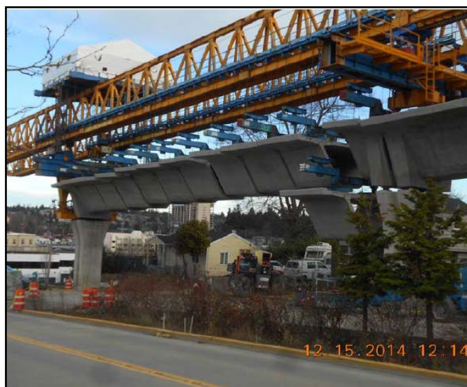
Gantry erecting span.
