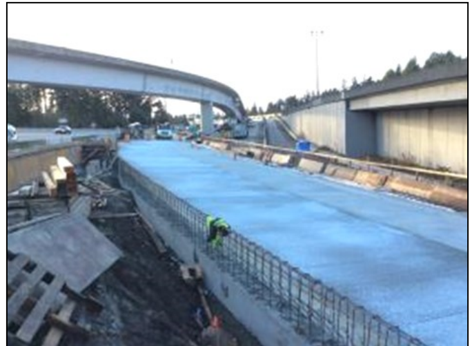
Paving the realignment of the Bellevue Way HOV off ramp from I-90.
