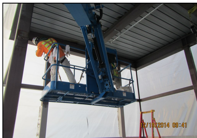
Painting the vent shaft roof.
