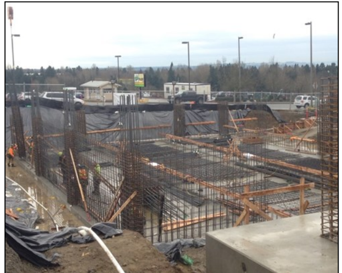
Workers placing columns and walls rebar at detention vault.
