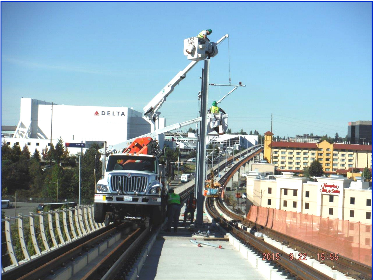
OCS pole installation—South 200th Link Extension
