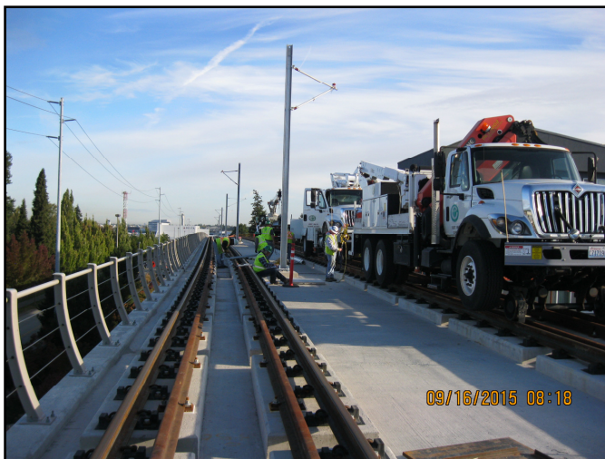
Cantilever arm installation on the guideway.
