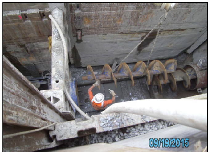
Completing installation of the 42" Casing at NE 100th St intersection with 1st Ave NE.
