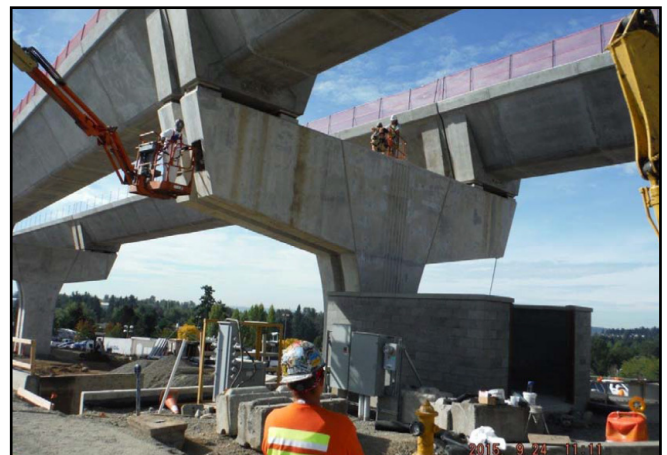
Grouting ongoing at T5 and T6 tendons.
