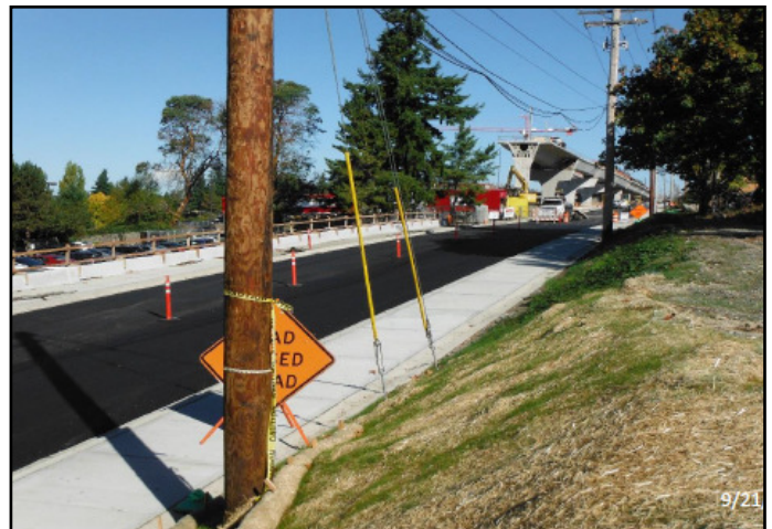
Looking north at 28th Avenue South Pavement.
