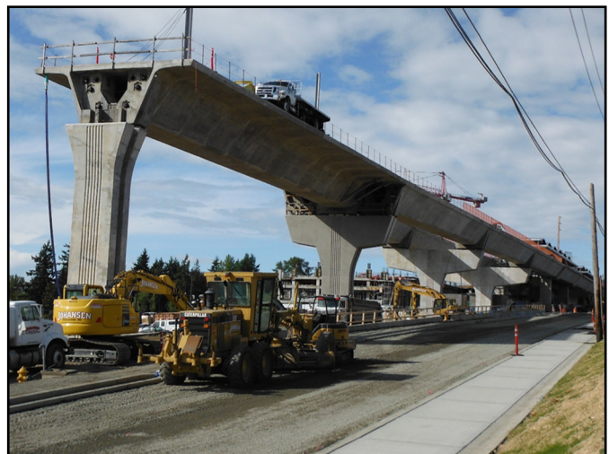
Prepping 28th Avenue South for paving activities.
