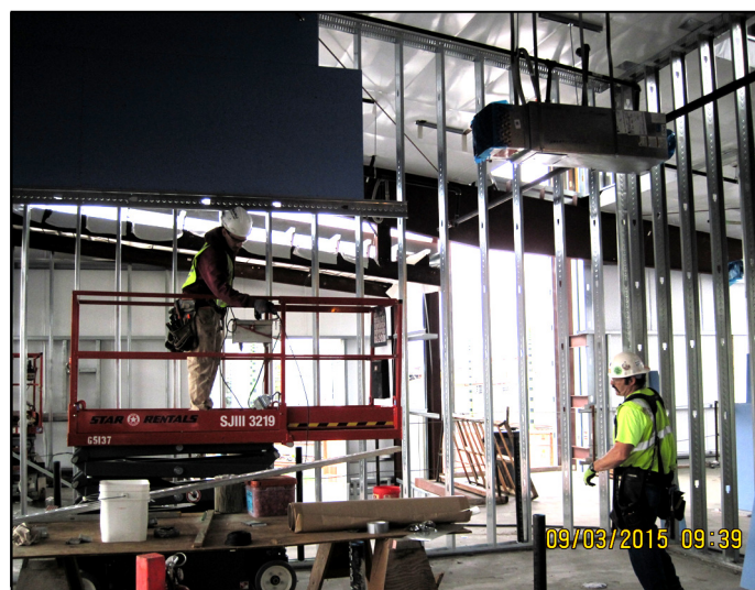
Installing wall board of 2nd floor.
