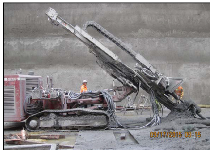
Drilling angled tie-backs for the thrust frame slab at south UDS shaft.
