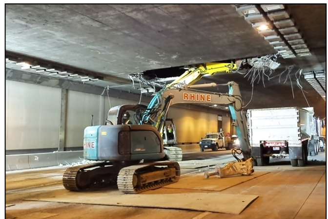
Demolition for ventilation improvements in the Mercer Island Tunnel.
