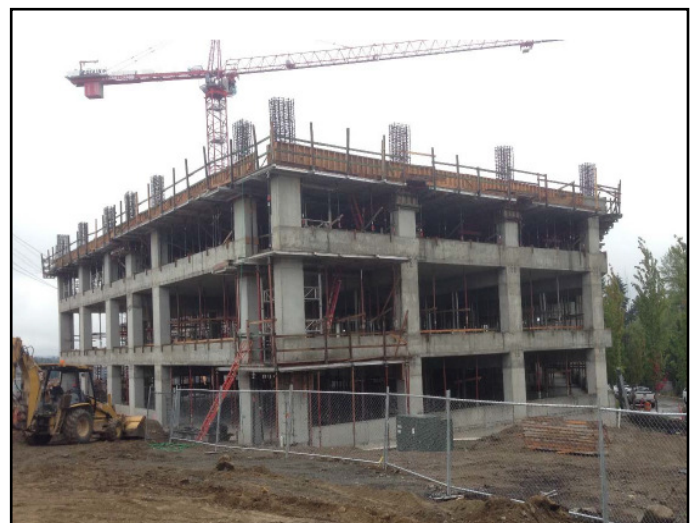
Elevated deck of Garage in place.
