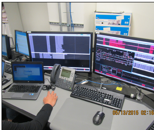
BMS testing at the OMF.
