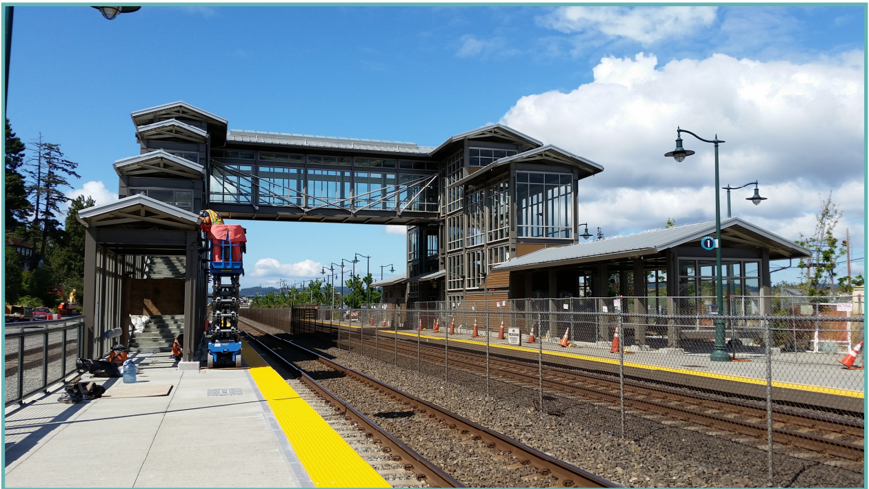
Completing downspouts and other final touches on the Mukilteo Sounder Program new platform.
