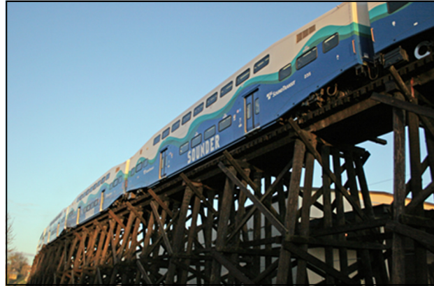
Project will replace existing Tacoma train trestle
