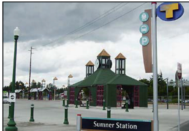
Improving access to Sumner Station
