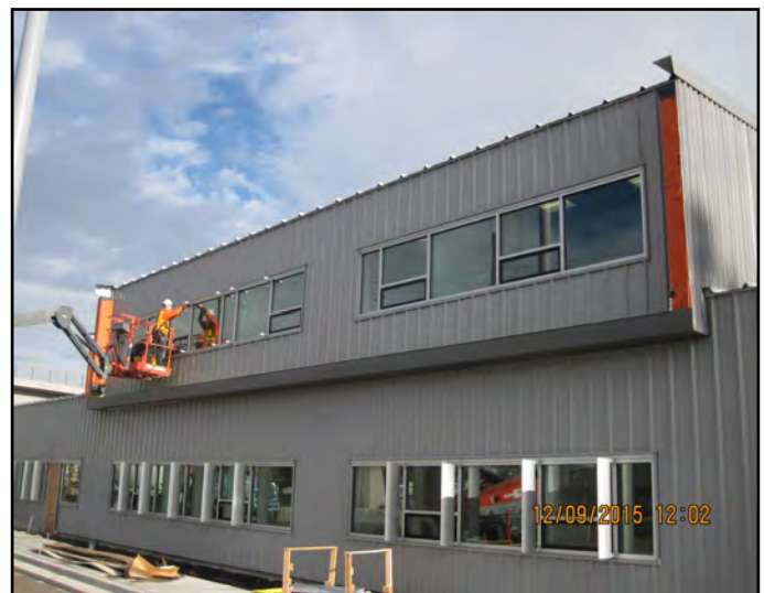
Continuing installation of sun shades.
