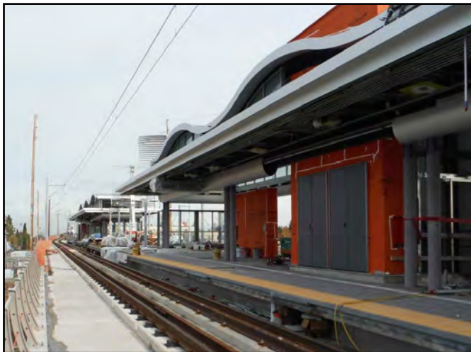
Progress north of Angle Lake Station.
