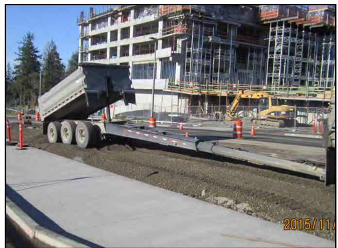
S. 200th Street activities ongoing-sidewalk and bus pull out work.
