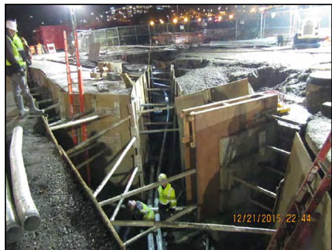
Duct bank work continues.
