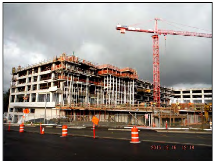
Parking garage structure as viewed from S. 200th.
