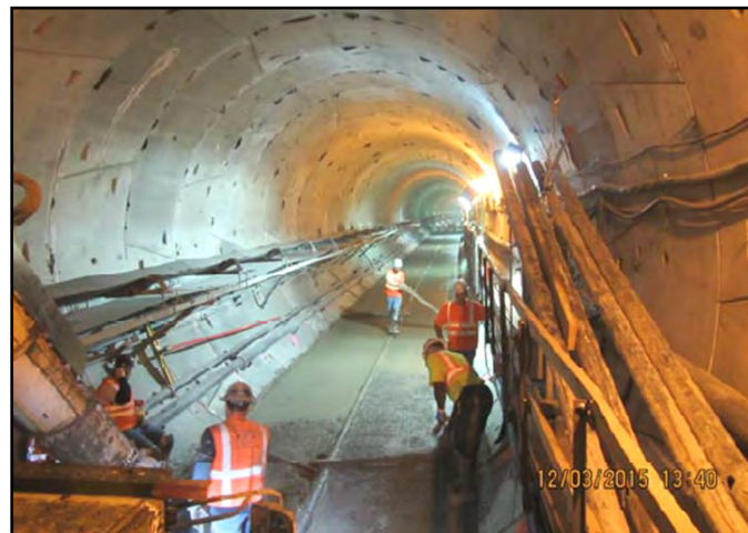
Pouring invert concrete for the NB tunnel from UDS to RVS.
