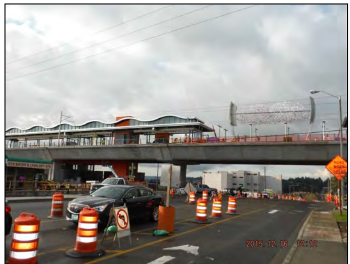
Looking west to the Angle Lake Station at the installed artwork.
