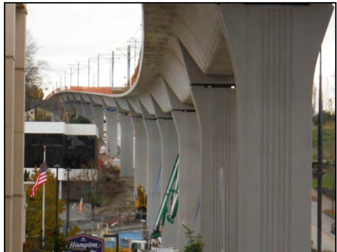
Guideway alignment looking south of Hampton Inn.
