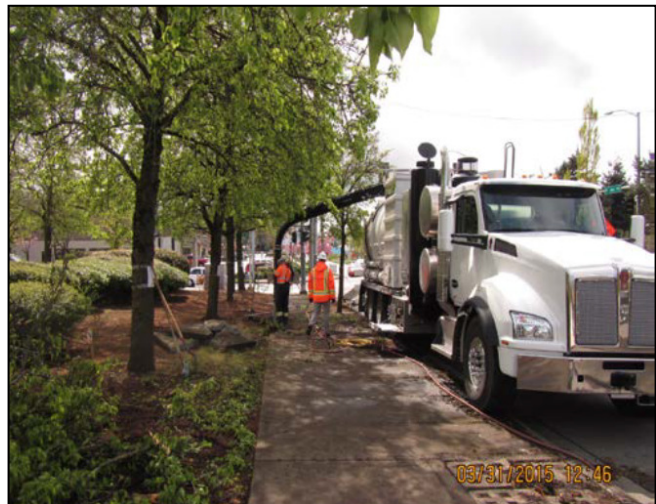
Contractor removing trees and verifying utility locations along the east side of 1st Ave NE from NE 100th to NE 103rd Streets.
