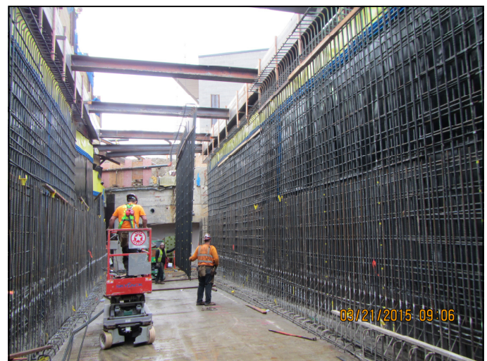
Workers working on rebar mat for walls of the pedestrian concourse.
