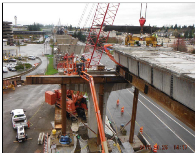
Erecting segments on falsework.
