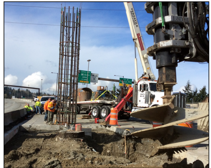
Construction crews setting the reinforcement cage for a sign bridge foundation on the R8A Stage 3A project.
