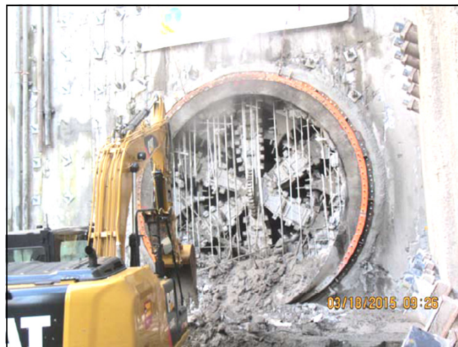
TBM No. 1 breaking through the north wall of RVS station box.
