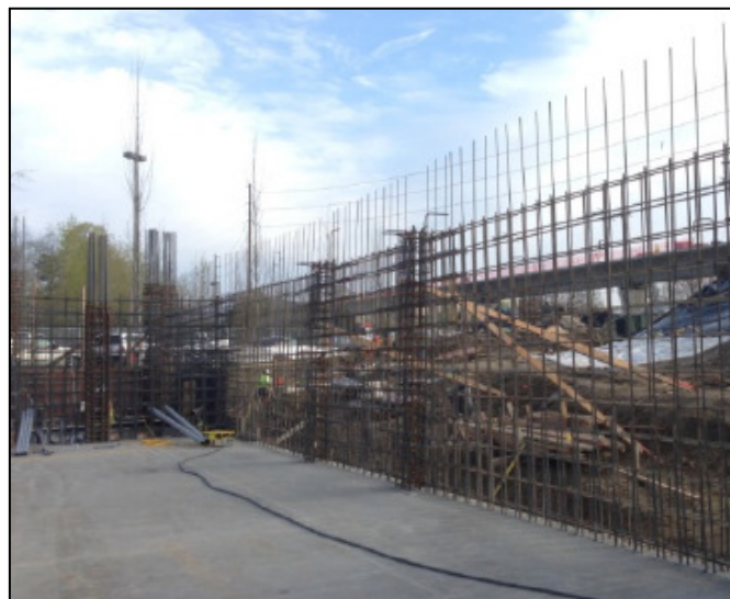
Rebar installation in progress for retaining wall between Level 2 & 3.
