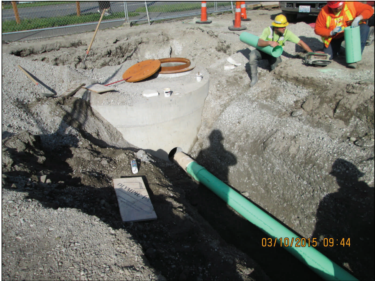
Mid-day Bus Storage installation of drainage connections to a stormfilter manhole.
