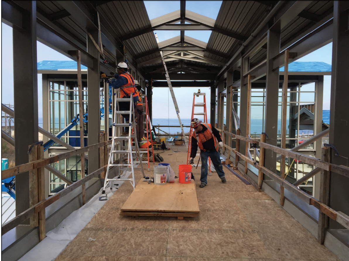
Setting window frames on bridge deck at Mukilteo Station.
