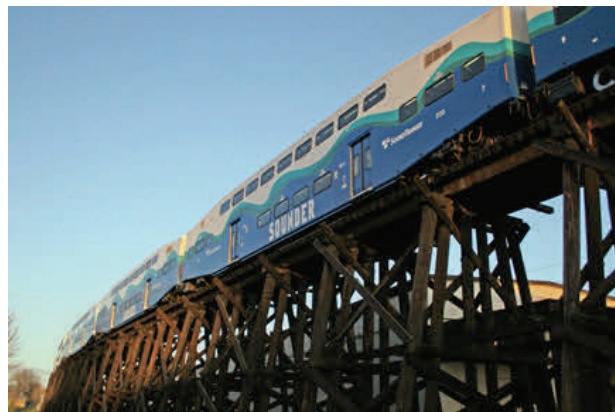
Project will replace existing Tacoma train trestle
