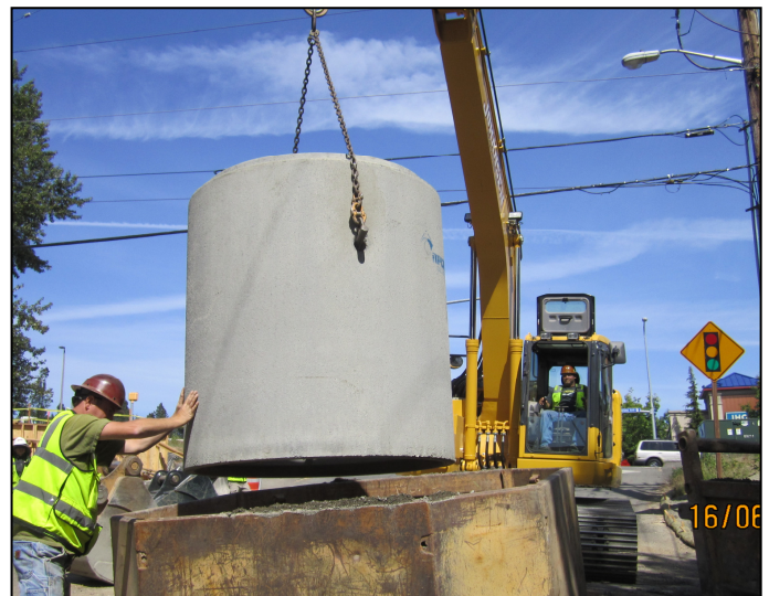
Installing a catch basin at 28th Avenue.
