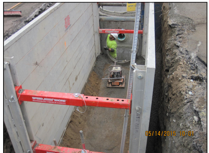
Advanced storm water utility relocation.
