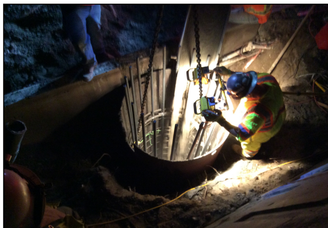
Contractor pouring a concrete shaft for a sign bridge foundation.
