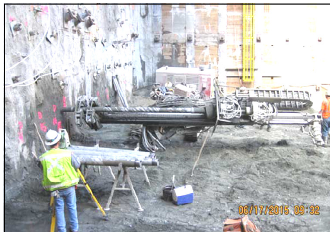
Drilling freeze pipe at south headwall of UDS shaft.
