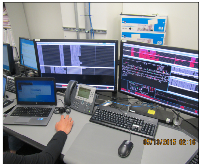
BMS testing at the OMF.
