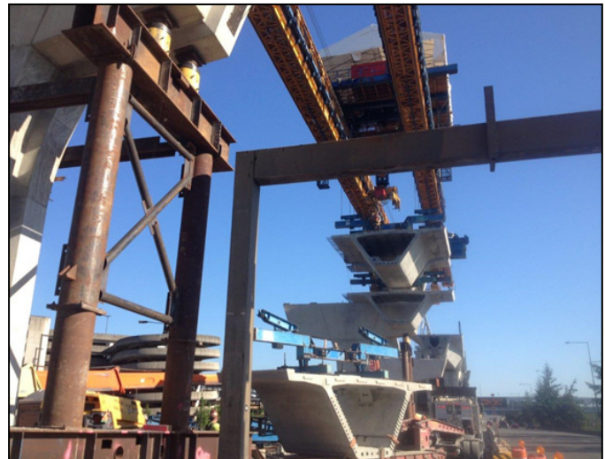
Segment installation at S440.
