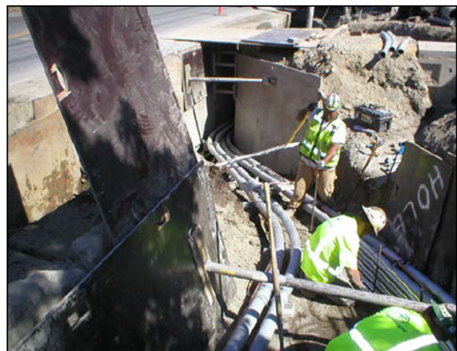
Ductbank construction and formwork installation
