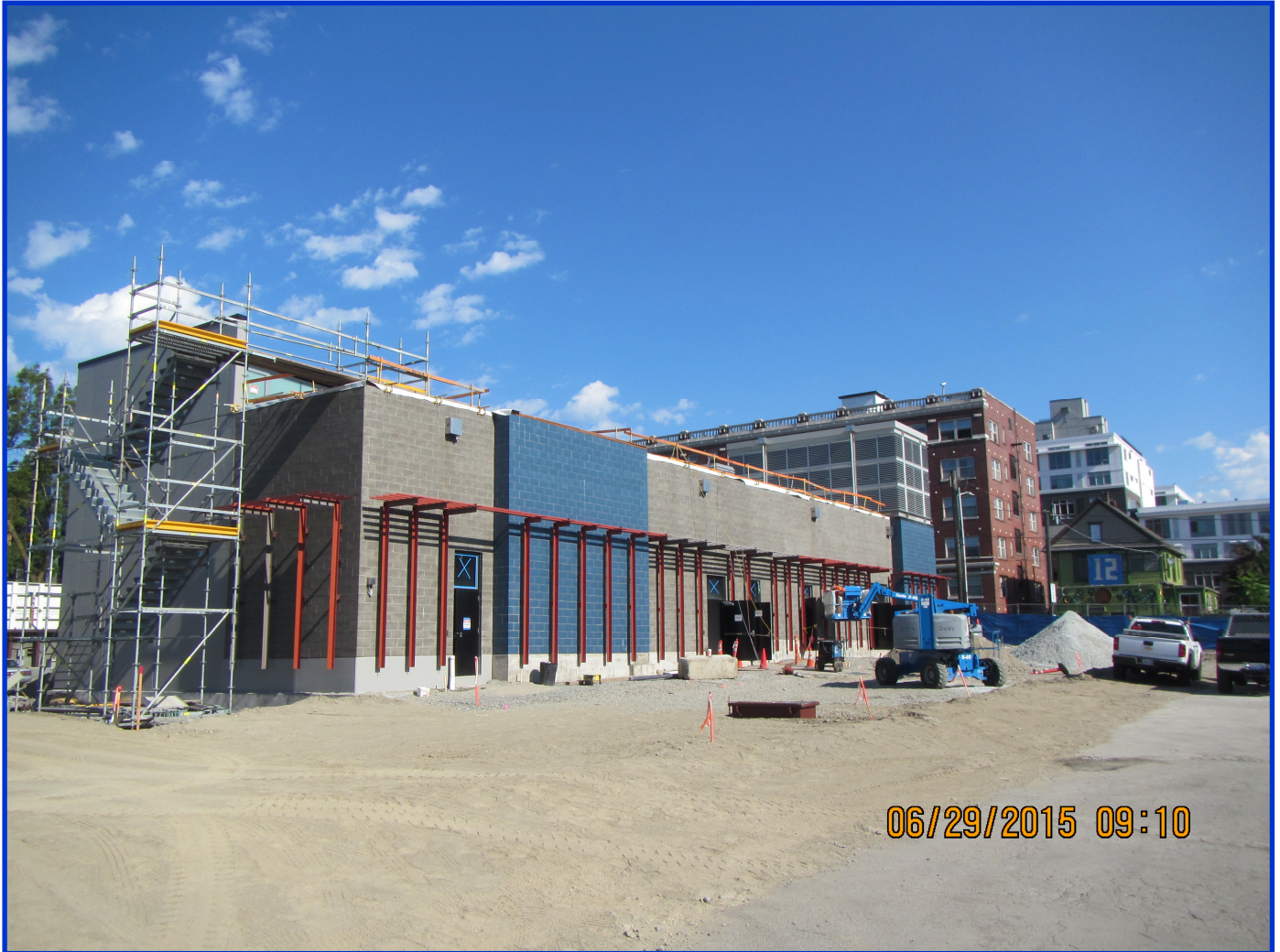
Overview of the north entry exterior of the Capitol Hill Station
