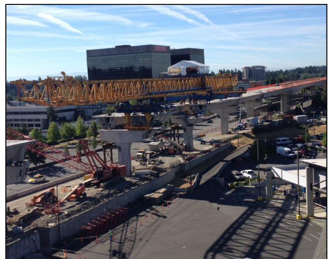
Preparing to begin with the segment erection.
