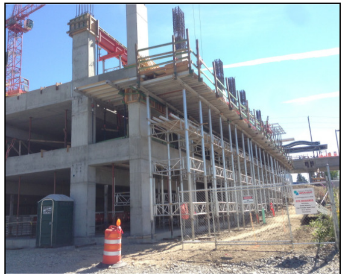
Forming in progress for Level 3 cantilever walkway of the garage.
