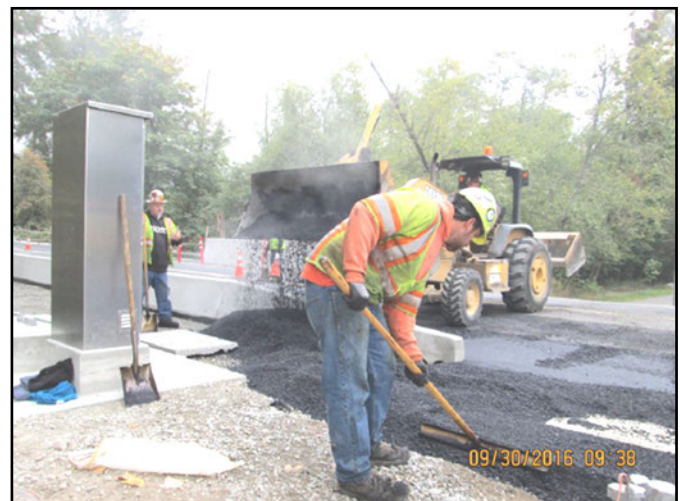
Paving at S. 200th Street– vicinity of Des Moines Creek.
