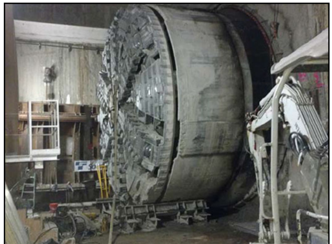
SB TBM front shield on cradle in UWS Retrieval Shaft.
