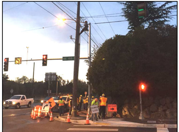
Potelco working with Seattle City Light during a night shift to coordinate permanent power connection for WSDOT signal.
