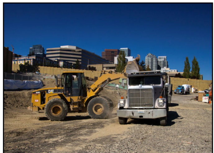
Excavation at the South Portal.
