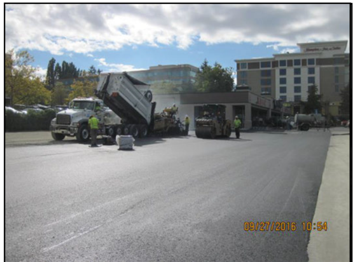
Installation of asphalt paving at parking lot.
