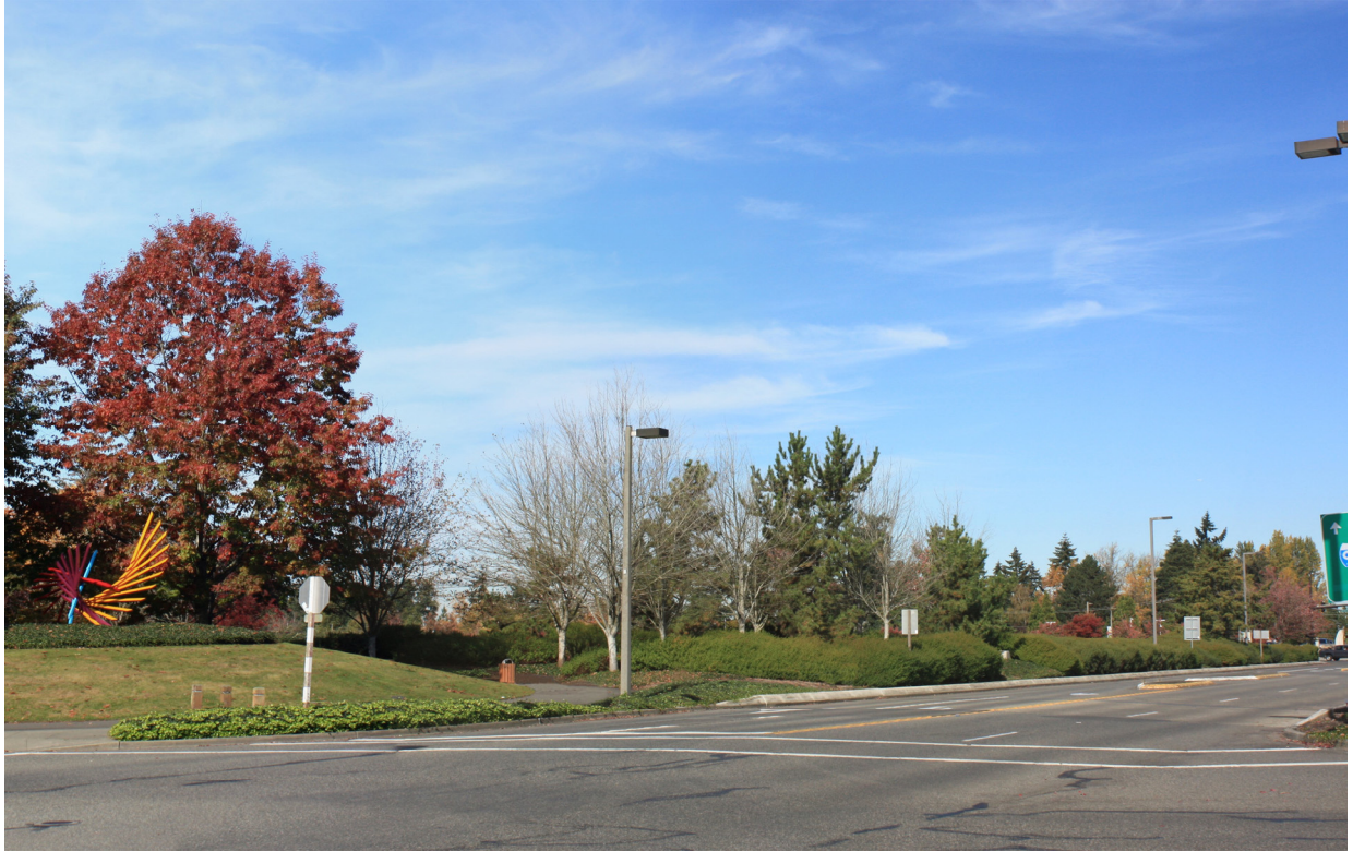
Exhibit 4-8. Existing Condition at Intersection of 80th Avenue SE and SE 27th Street – Looking Northwest from Sidewalk
