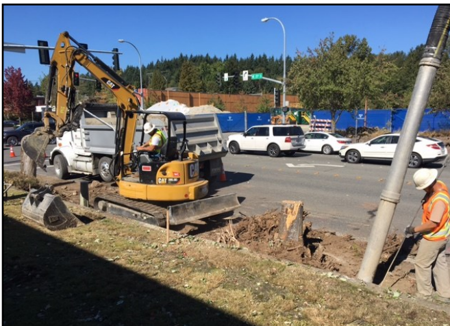
Excavating for new PSE vaults
