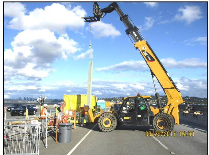
Ongoing work on I-90—workers lowering beam into hatch of pontoon.
