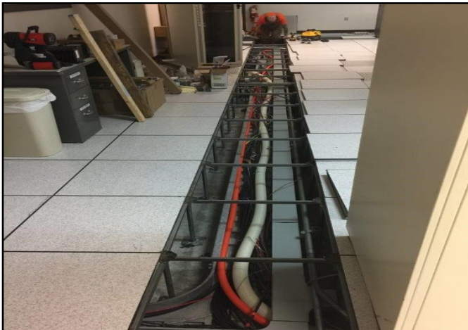
Concealed Communications Wiring Installation
