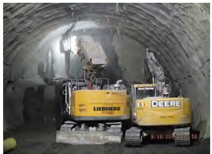
Excavating tunnel top heading in the Downtown Bellevue Tunnel.
