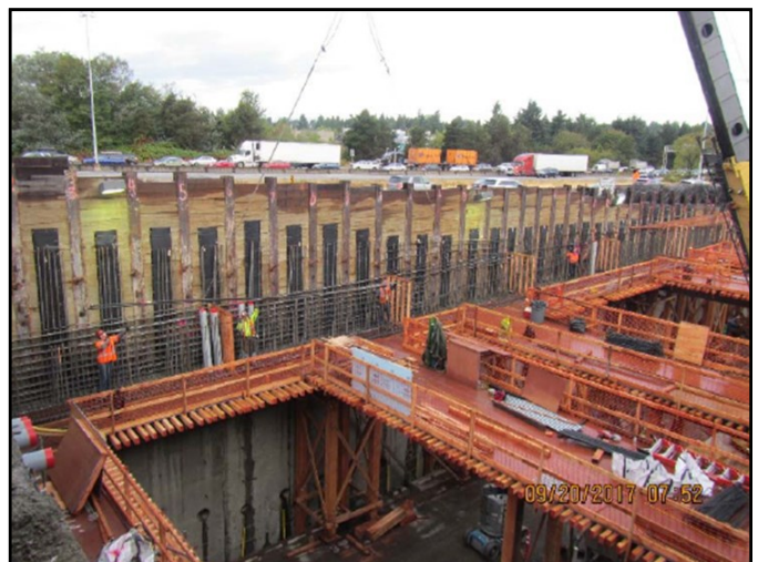
MLP: Setting up waler rebar above west wall of portal structure.
