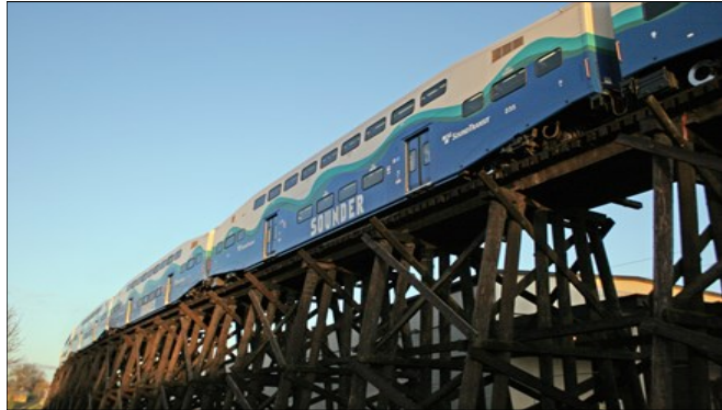
Project will replace existing Tacoma Trestle
