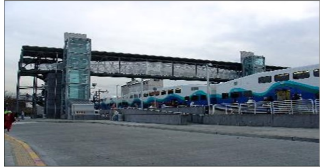
Improving access to Kent Station
