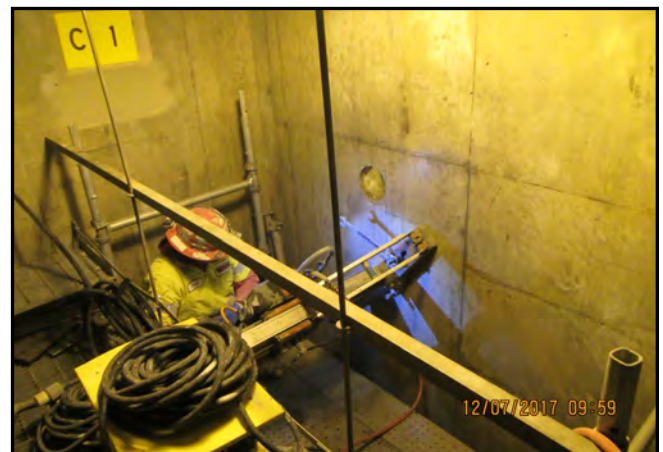
Coring interior pontoon wall for post-tensioning strand installation.
