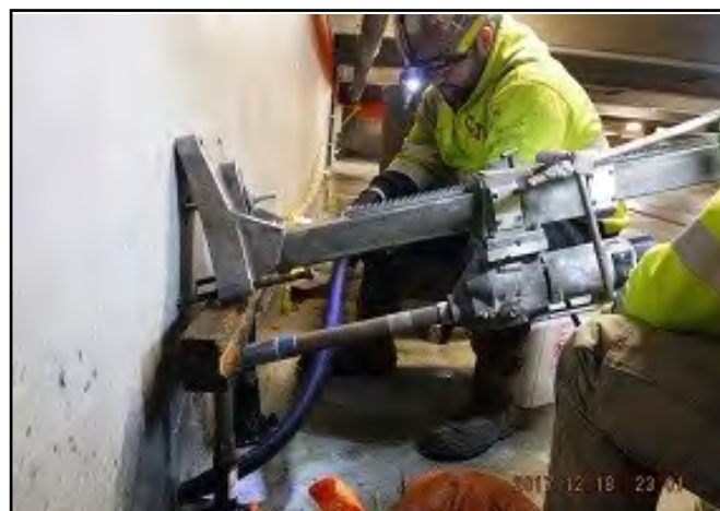
Skyline Garage void grouting ongoing.
