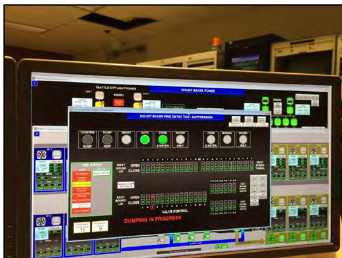
Testing fire zone systems in Mt. Baker Ridge Tunnel Control Room
