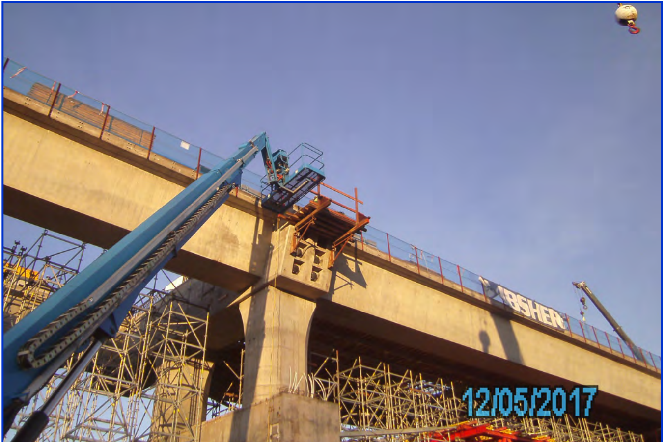
Building the deck for the overhead catenary system formwork at the track slab (Northgate Link Extension)
