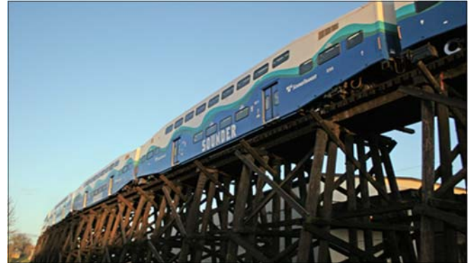
Project will replace existing Tacoma Trestle
