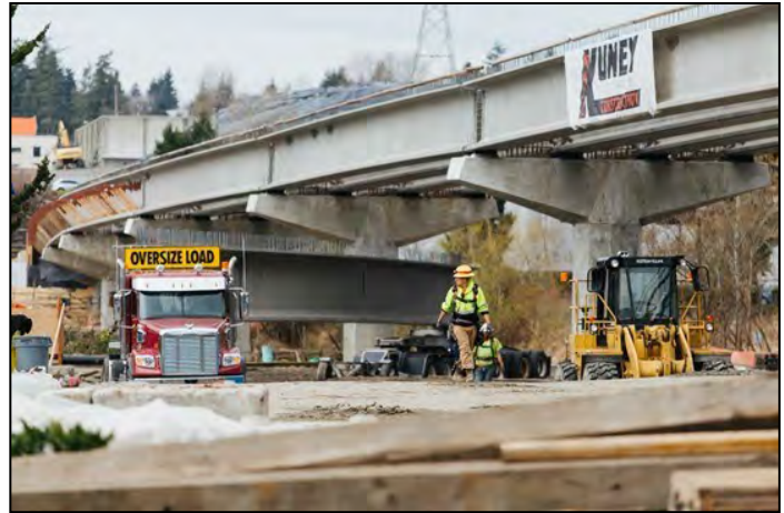
Bel-Red girder set for aerial guideway.
