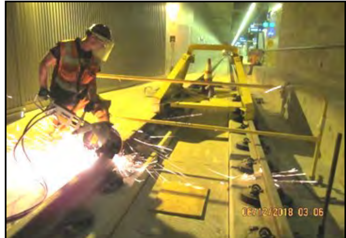
Trackwork crew cut rail for installation on the floating slabs in the NB tunnel.
