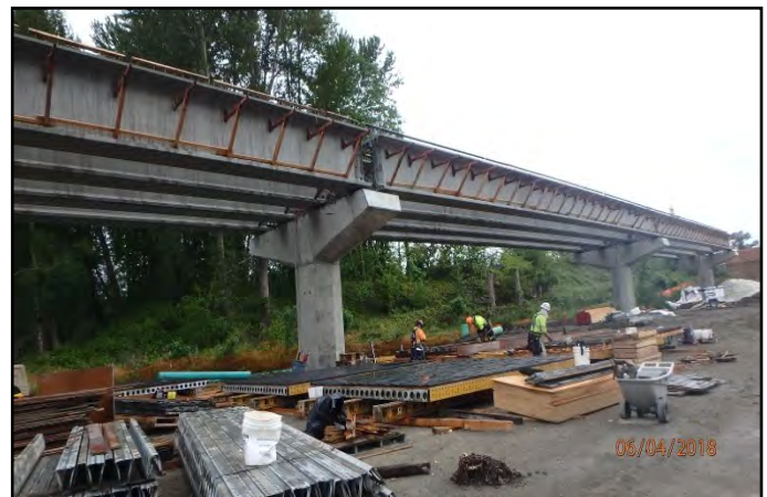
Bridge Crew resumed fabrication of abutment wall concrete
