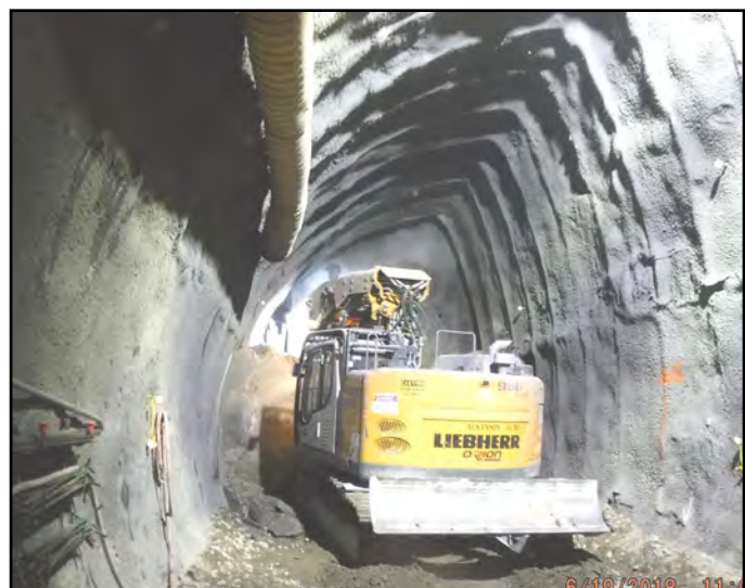
Tunnel excavation top heading.
