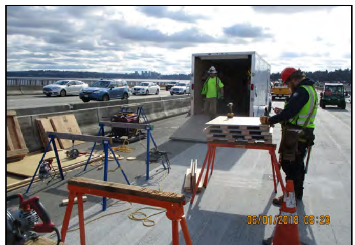
Fabricating forms for transverse PT anchorages on Pontoon F and O.
