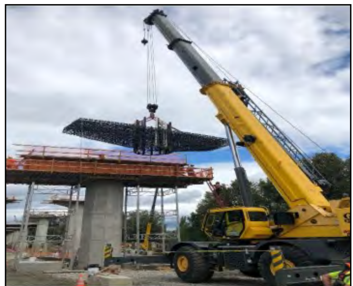
Installation of cage pick on I-90 guideway.
