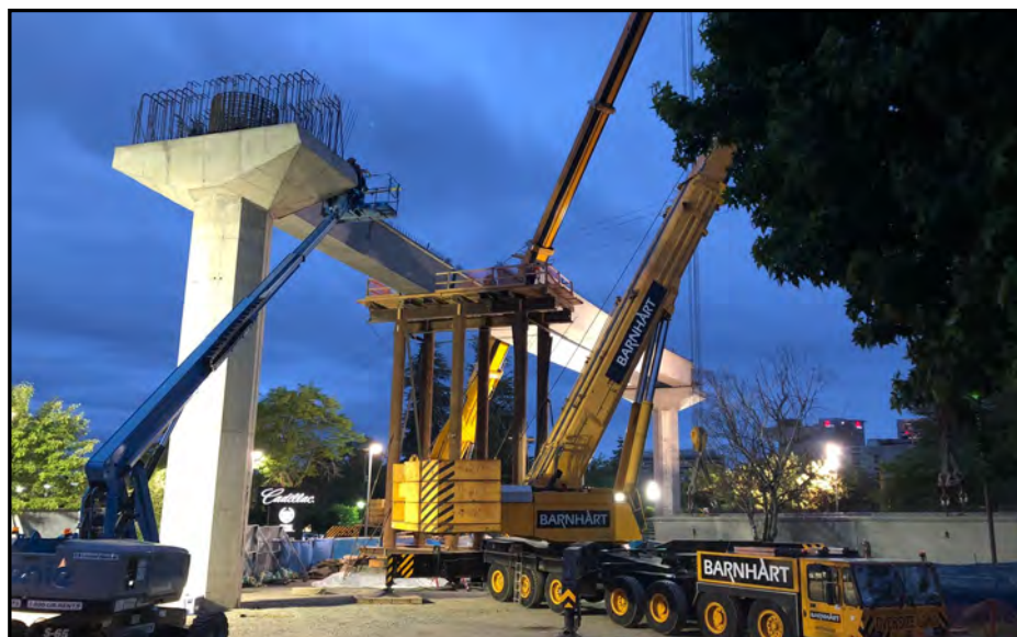
E335 Downtown Bellevue to Spring District: Rigging of girder during NE 8th St. closure.
