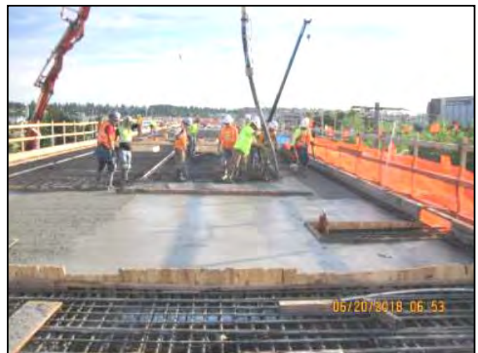
Placing concrete for deck span A05 Guideway looking north.
