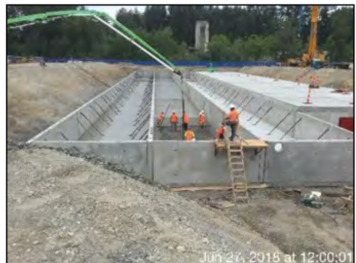
Vault "A" sloped floor placement.
