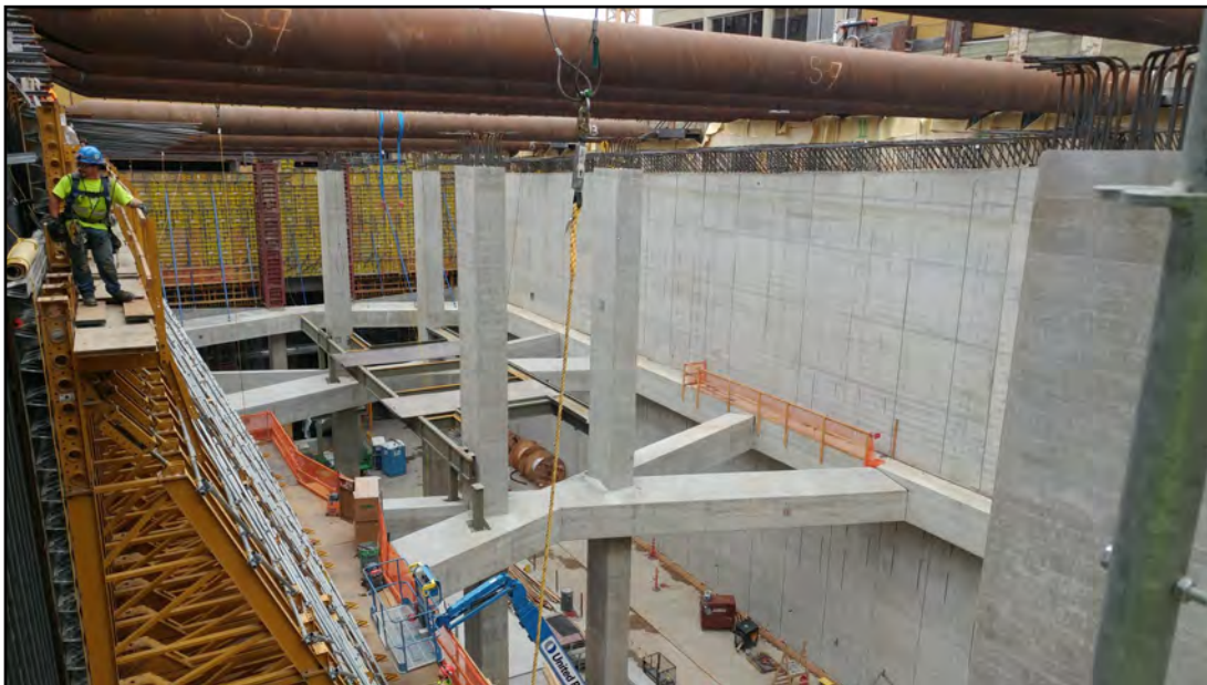
N140 Station box with structural cross-bracing at Mezzanine level —view to the south.
