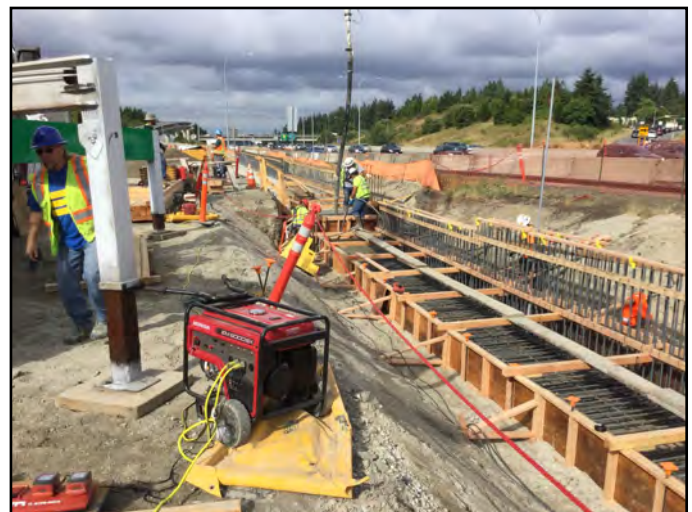
Overlake Village Station sound wall footing FRP.
