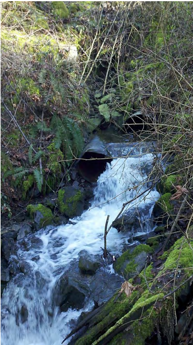
Redondo Creek exiting the culvert under the utility corridor drive. This culvert poses a fish passage barrier.
