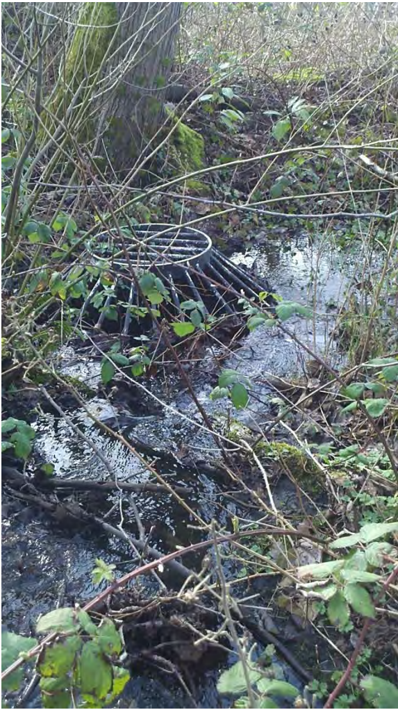
Vertical drain at the west end of the Massey Creek reach in the study area. This structure conveys the creek into a pipe system under an apartment complex and roadway and poses a complete passage barrier to fish.
