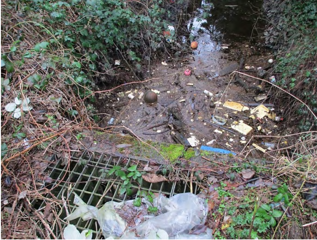
Bingaman Creek trash rack at culvert entrance on south side of S 288th Street.
