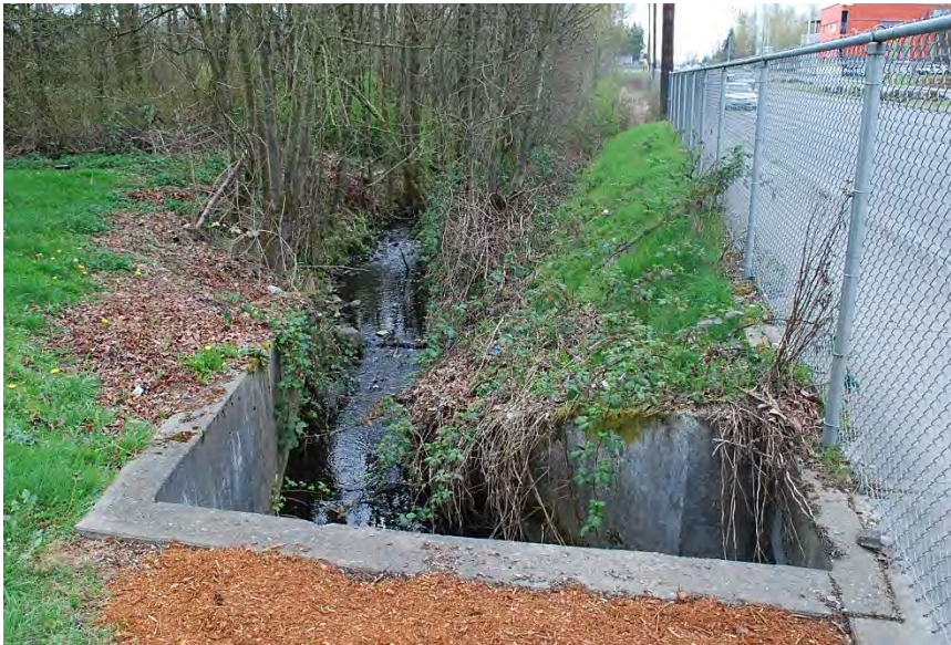
McSorley Creek alongside SR 99 where it enters a 4-foot-wide concrete box culvert under the highway.
