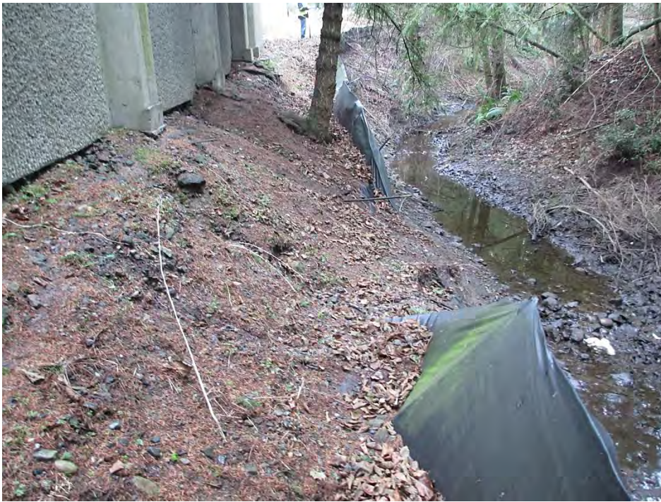
Bingaman Creek right bank eroding next to sound wall along Bingaman Creek reach south of S 288th Street.
