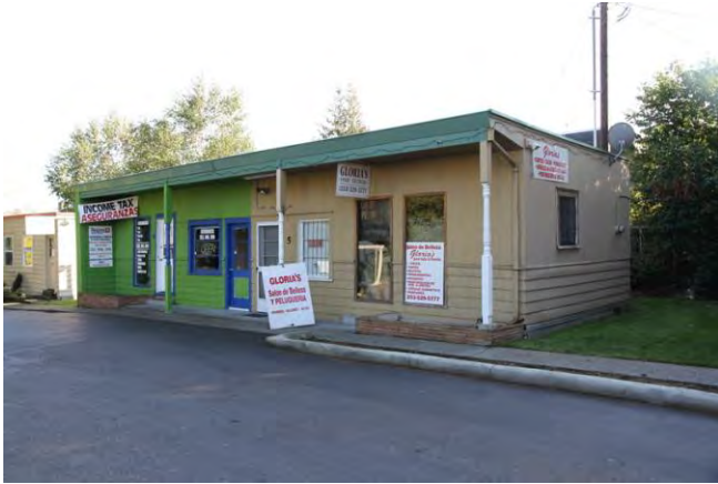
Northwest corner, south row, building 3 2013
