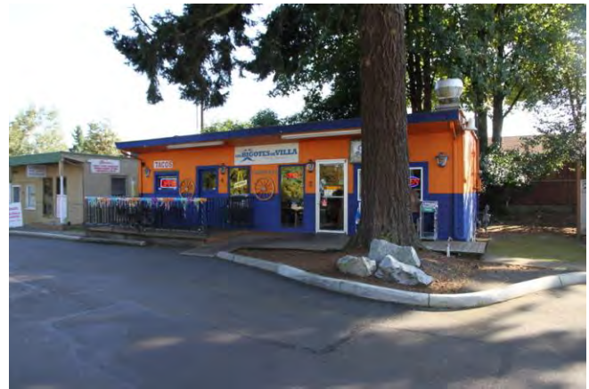
Northwest corner, south row, building 2 2013
