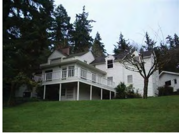
Courtesy of King County Assessor's website. Northwest corner 2013
