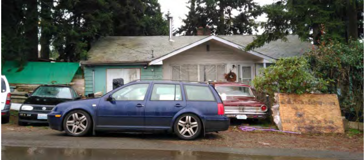
Photo 1. 2947 S 252nd Street Front (north) elevation
