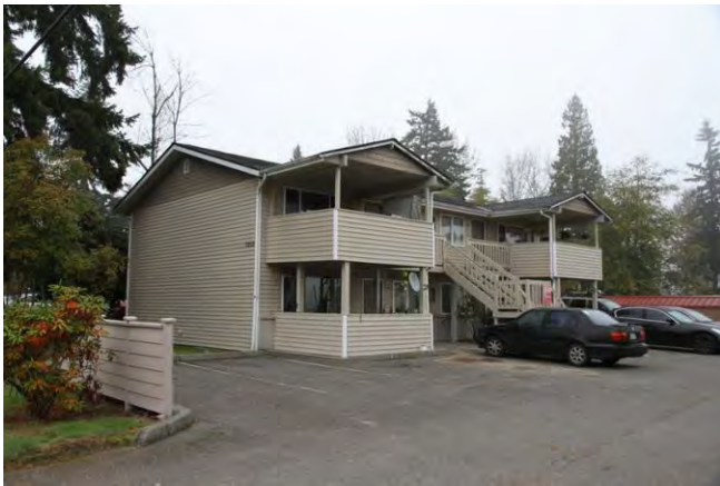
Southwest corner, north building 2013
