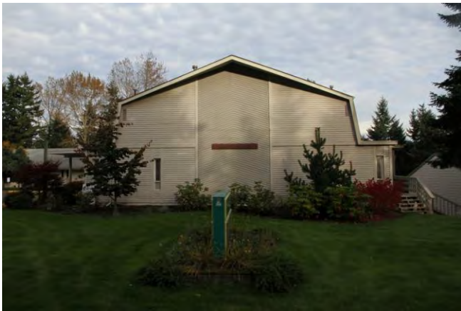
West elevation, west wing 2013
