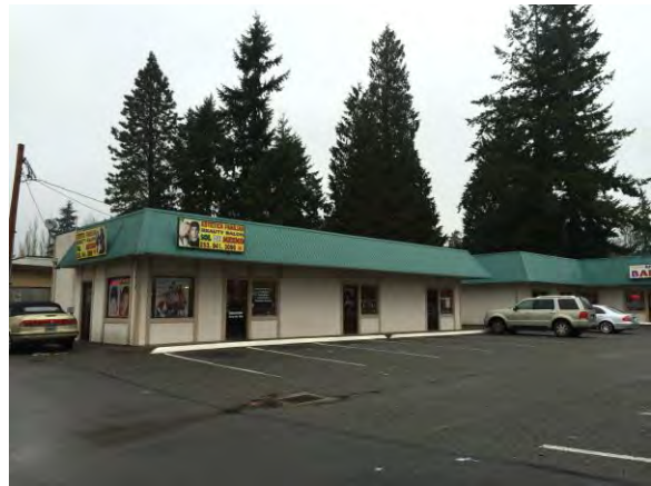
Southwest corner, 1976 building 2013
