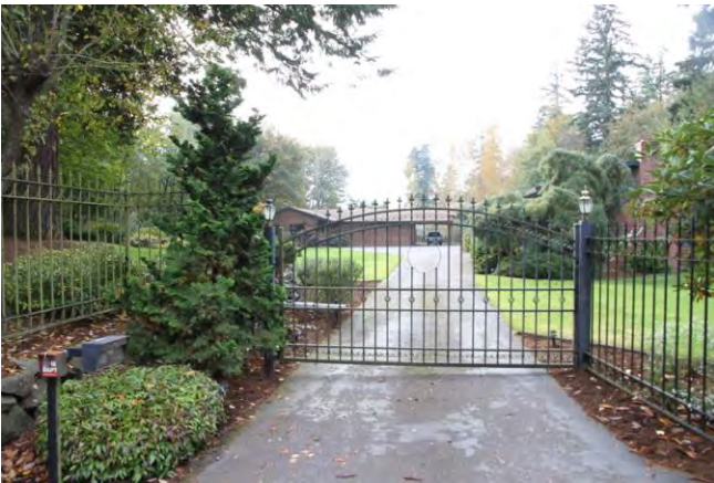
View west, includes detached garage building 2013
