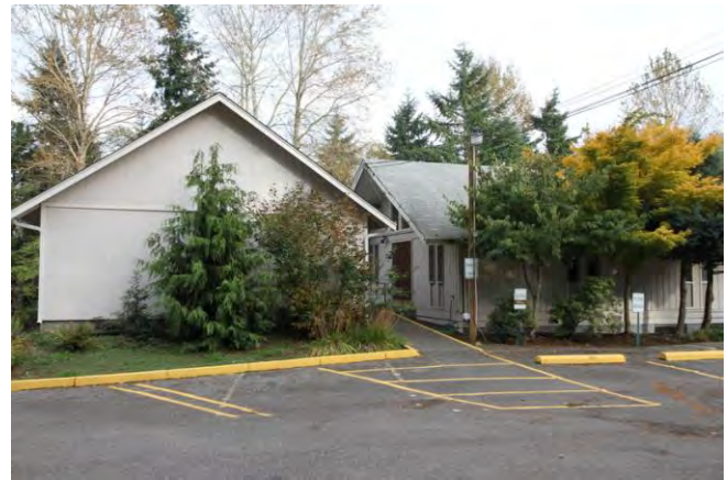
Northwest corner (north wing), west elevation (2009 shed) 2013
