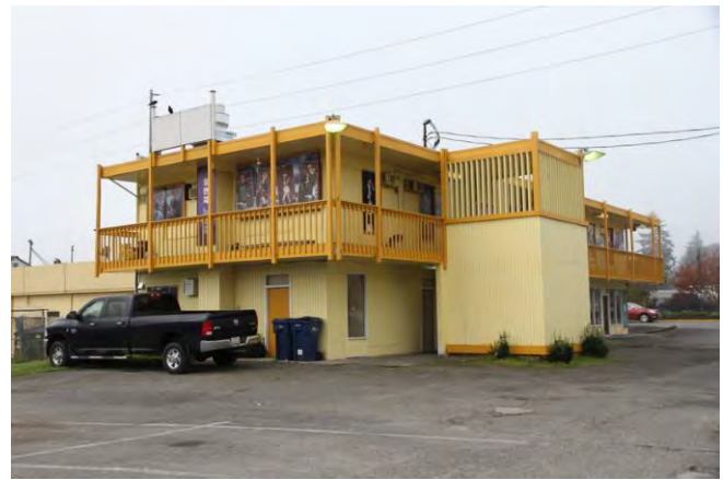
Northeast corner, 1960 building 2013
