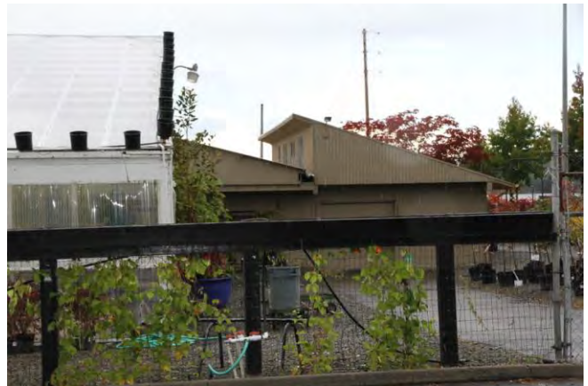
1968 retail section on the right, greenhouse on the left. South elevation, east end 2013
