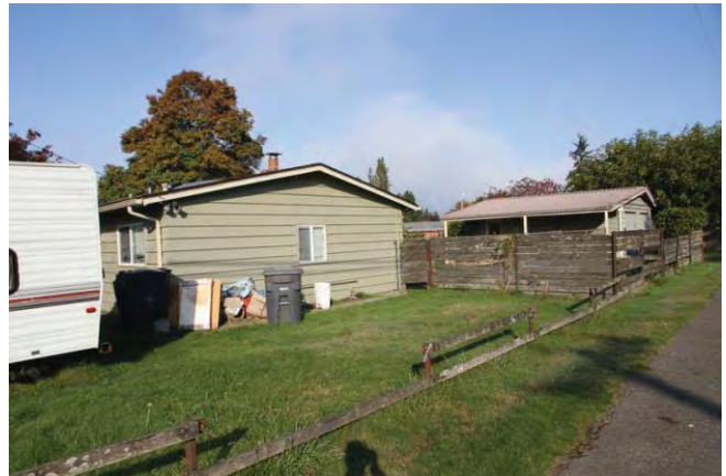
East elevation, with detached 1960 garage addition 2013
