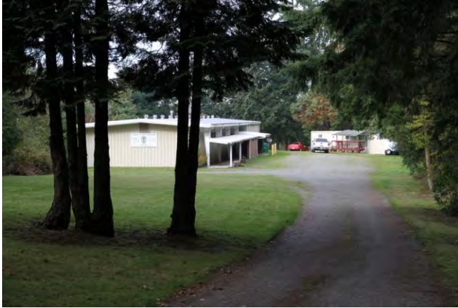
Southeast corner, trailer building visible 2013
