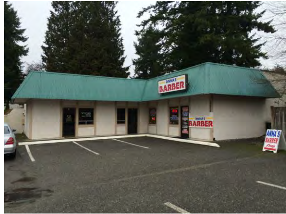
Southwest corner, 1980 building 2013
