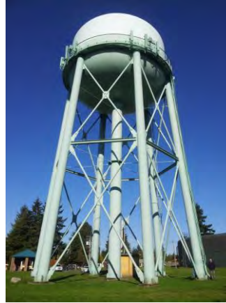
1958 water tower View to the north 2014
