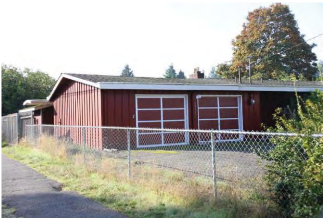
Northeast corner, second interior garage addition 2013
