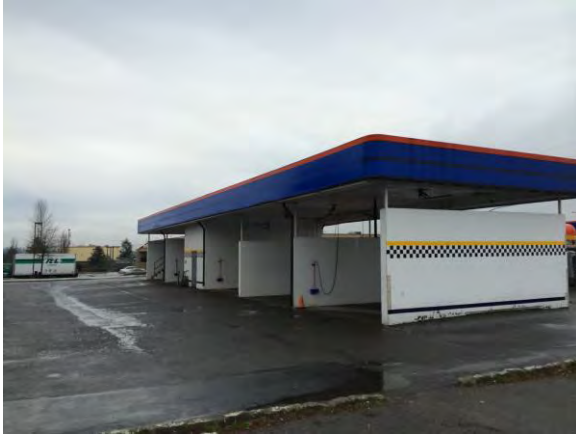
Northeast corner, 1970 structure 2014
