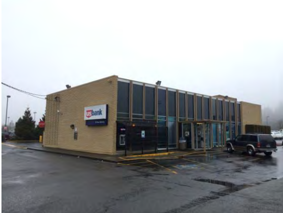
ATM enclosure addition is visible near center of photo Southwest corner 2013
