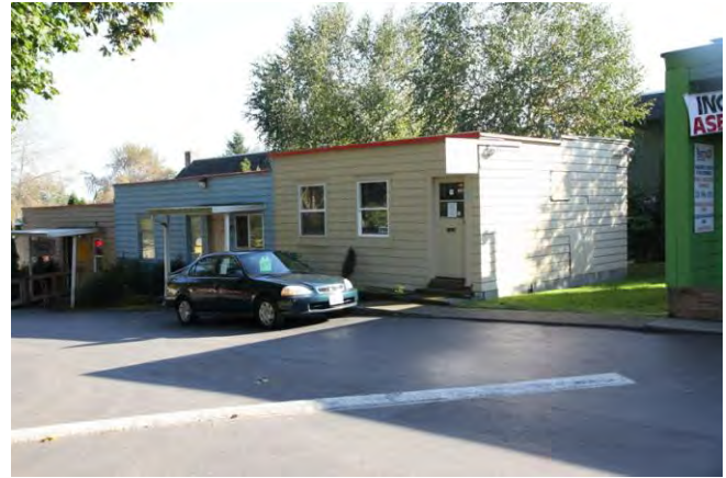
Northwest corner, south row, building 4 2013
