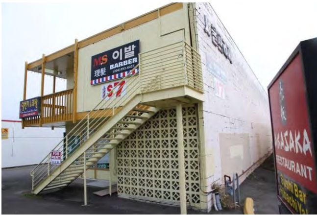
Southwest corner, 1960 building 2013
