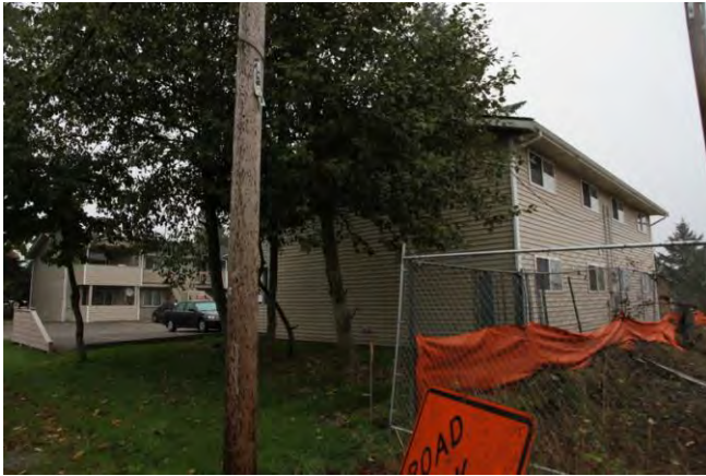
Southwest corner, south building 2013
