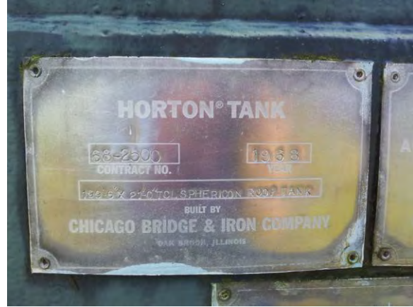
Label on 1968 water reservoir, detail 2014
