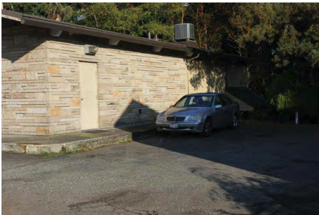
East elevation, view to the northwest 2013
