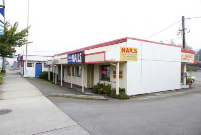
Southwest corner, 1947 building 2013
