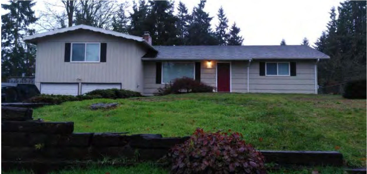
Photo 2. 2819 S 299 Place Front (north) elevation
