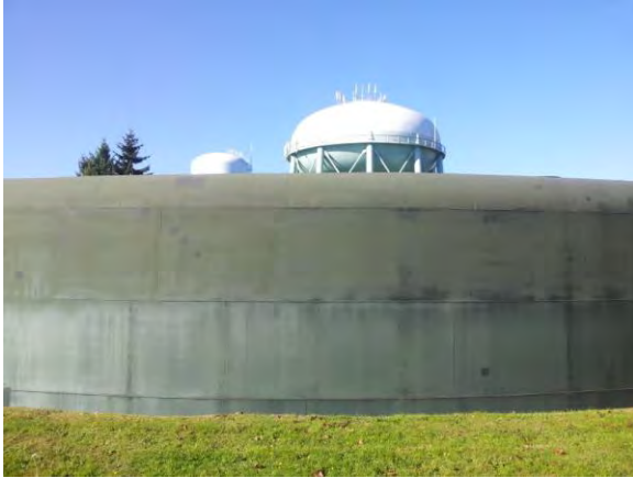
1968 water reservoir View to the west 2014
