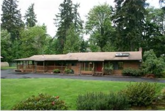
Photo courtesy of the King County Assessor's website. South elevation 2013
