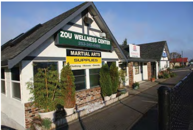
East elevation, view to the northwest 2013
