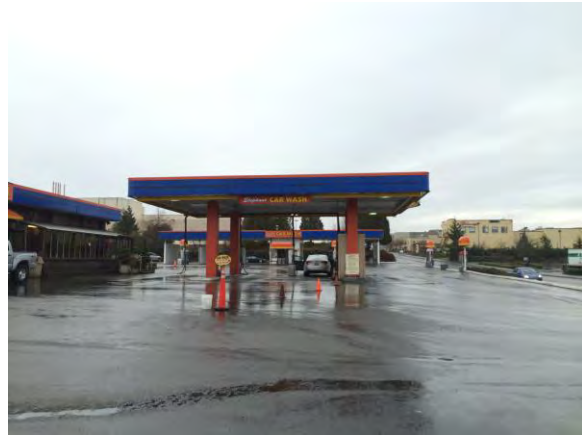
West elevation, 1980 canopy 2014
