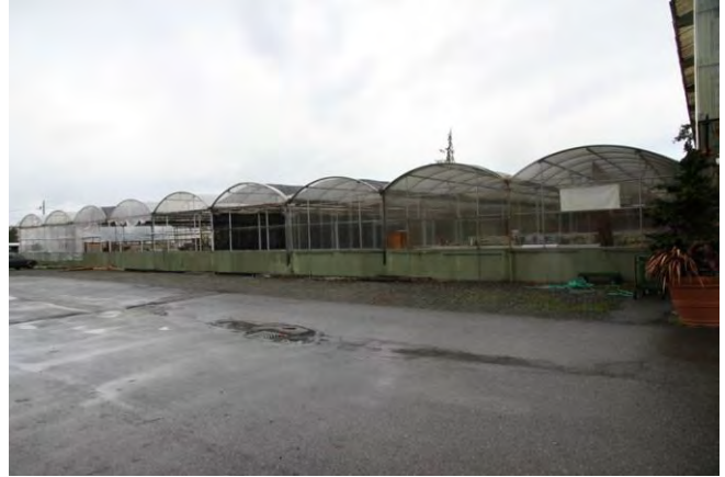
Barrel-roofed greenhouses at the west side of the property. South elevation, view to the northwest 2013
