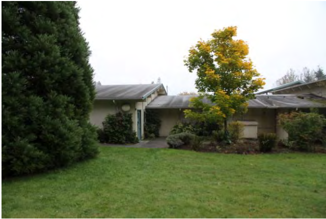
West elevation, further north 2013
