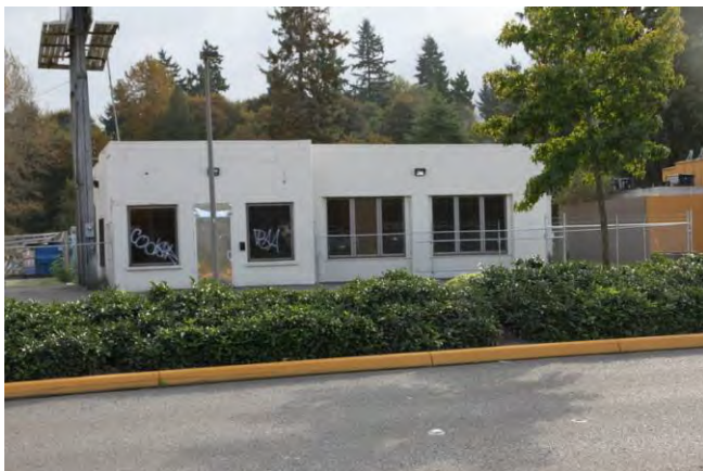
The two former garage door openings that are now two sets of three windows are on the left. West elevation 2013
