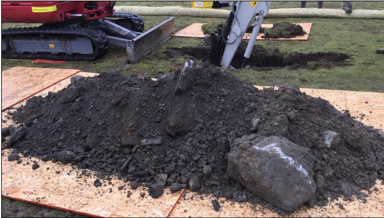
Figure 5 Typical fill material containing concrete and modern debris.
