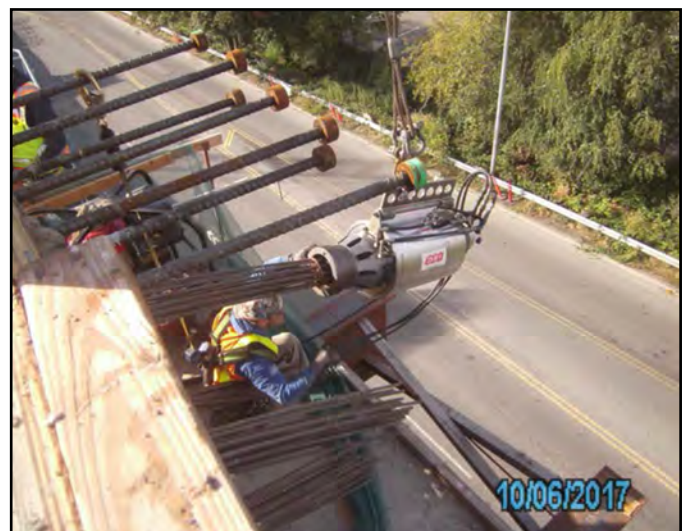
Stressing multi-strand tendons at C1 platform cap.
