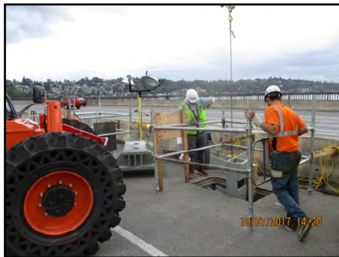
Lowering anchor supports through hatch in Pontoon E at I-90.
