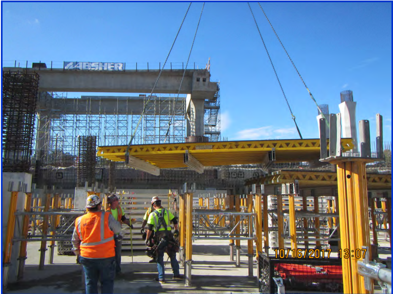
Setting deck forms at the Northgate Station
