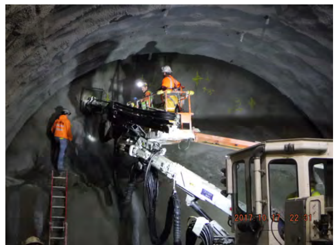
Probe drilling at tunnel top heading in the Downtown Bellevue Tunnel.
