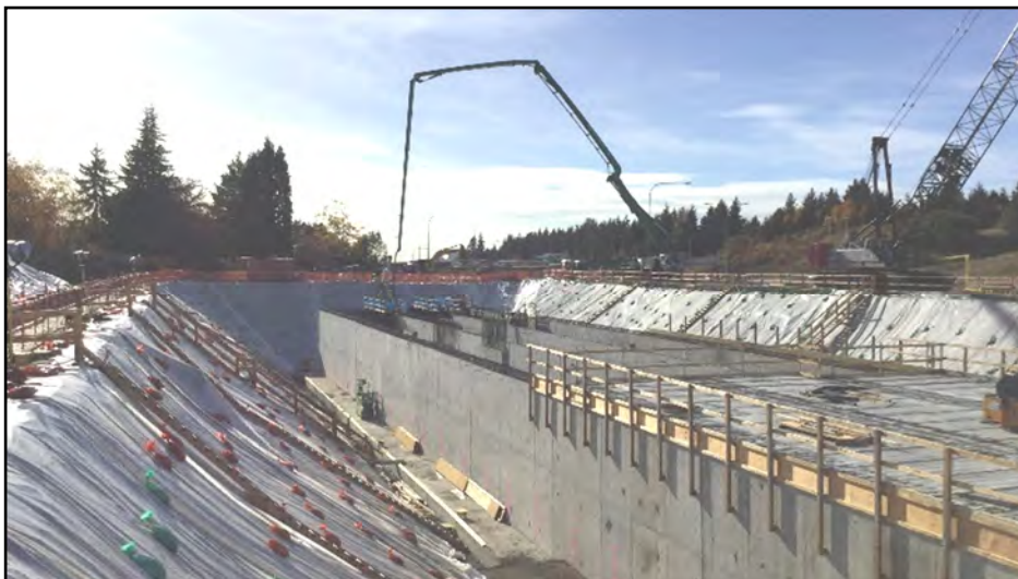
OVS Infiltration Vault CIP Wall Placement
