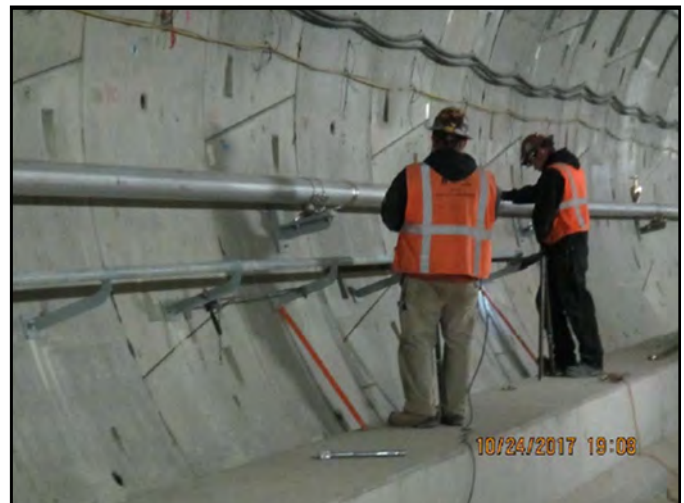
Installing tunnel handrails in the NB tunnel.
