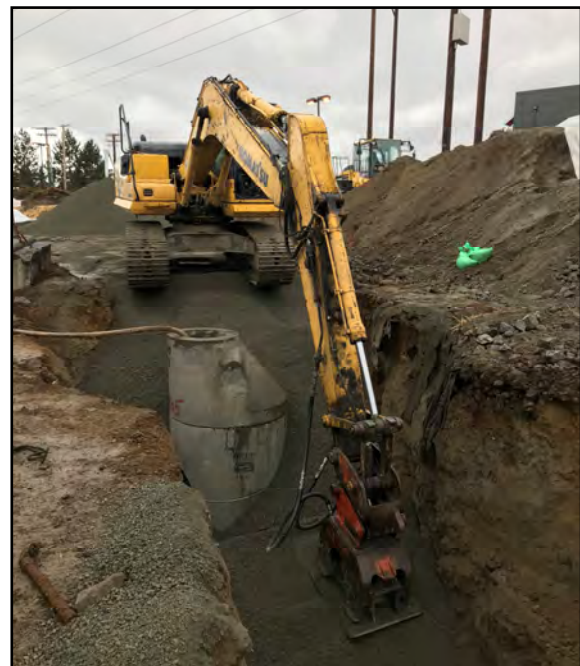
Backfilling trench
