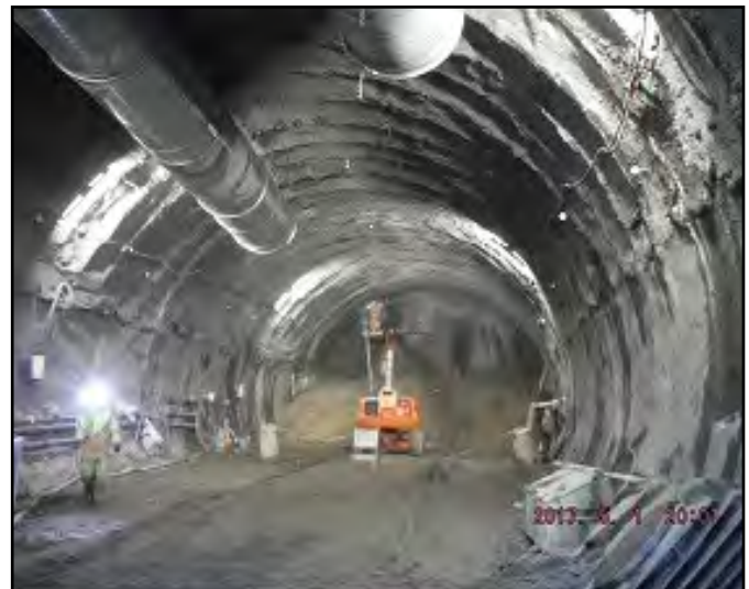
Tunneling advancing, excavation ongoing.
