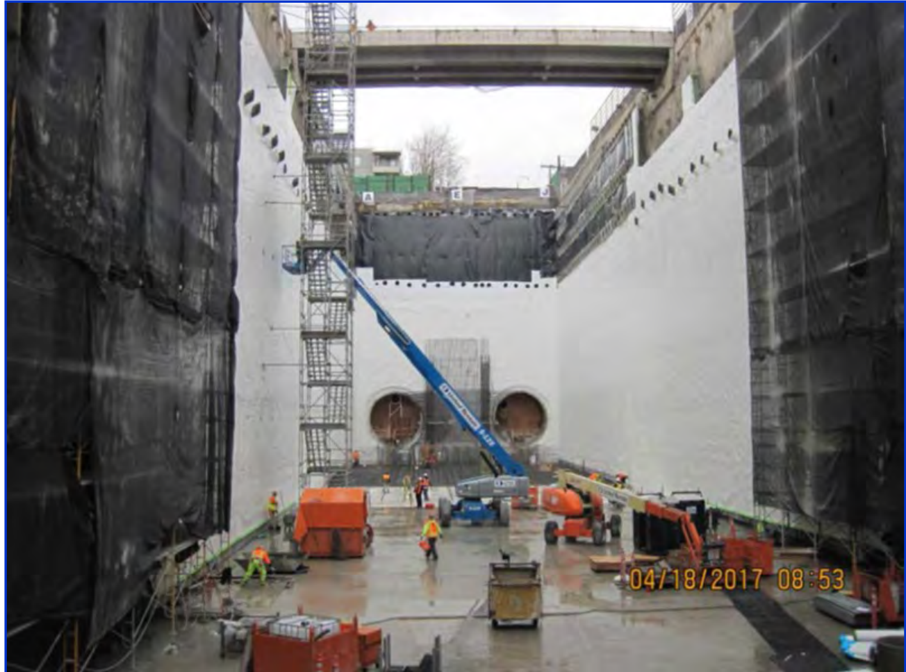
Northgate Link - Waterproofing activities at the Roosevelt Station
