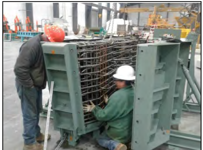
CPP workers assembling formwork in their facility.
