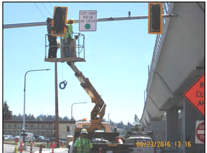
Installing traffic signals at S. 200th.
