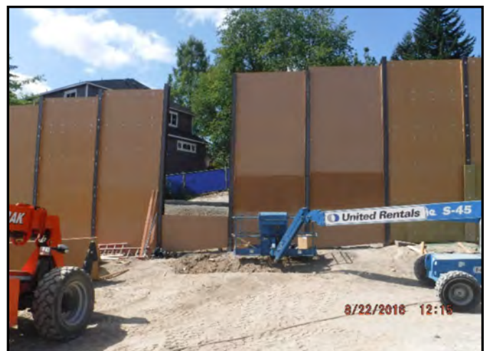
Sound wall panels closing off hammerhead area.
