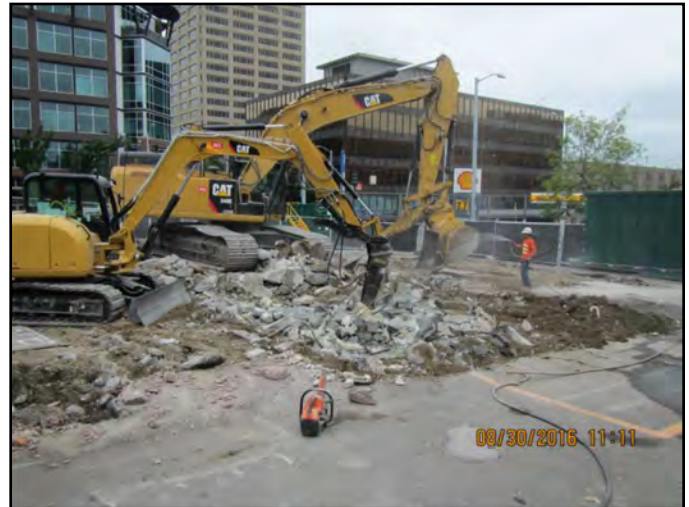
Demolishing building foundation at Key Bank site.
