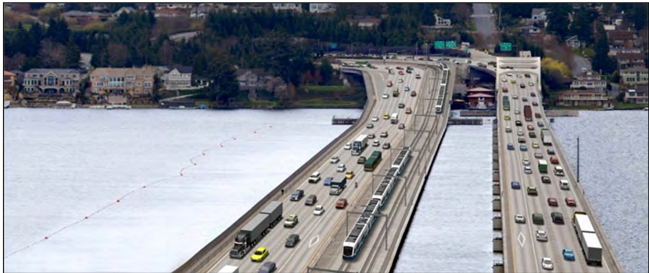
The project, when completed, will enable 24/7 HOV access on I-90 between Seattle, Mercer Island and Bellevue.
