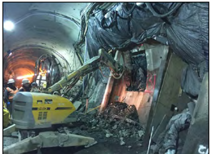
Breaking through NB tunnel segments at CP31.
