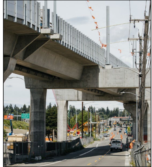
Figure 2-32 Straddle Bent
