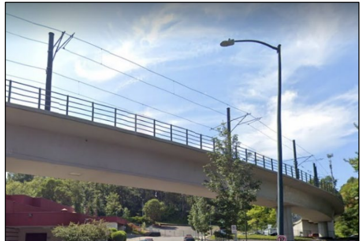
Figure 2-2 Typical Overhead Catenary System
