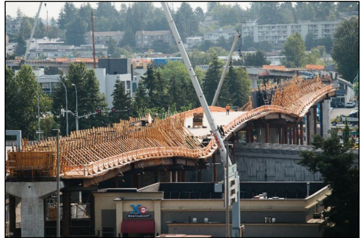
Figure 2-37 Construction of an Elevated Guideway
