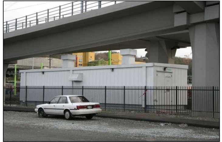
Figure 2-3 Traction Power Substation
