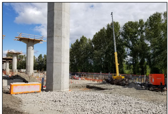
Figure 2-39 Construction of Guideway Columns
